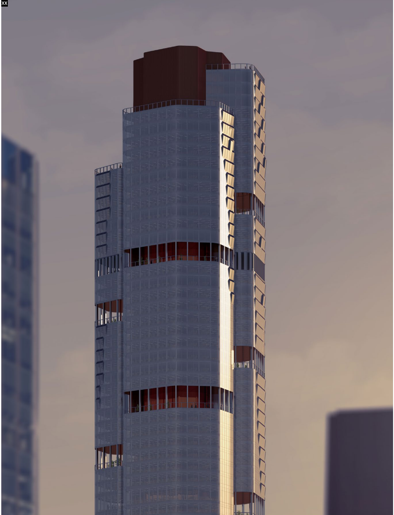
Fig 27: Exterior view showing an agglomeration of facade conditions.
