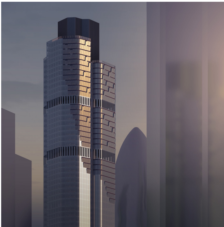
Fig 22: Introduction of a photovoltaic array - before and after.
