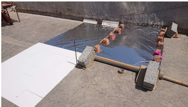
Figure 31: Field Experiment of Different Roofing Treatments for Horizontal Concrete Slab Roofing
