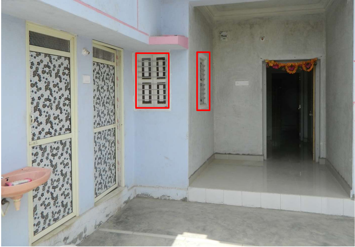
Figure 37: Front view of the as-built Bhuj housing (Kitchen windows highlighted in red)
