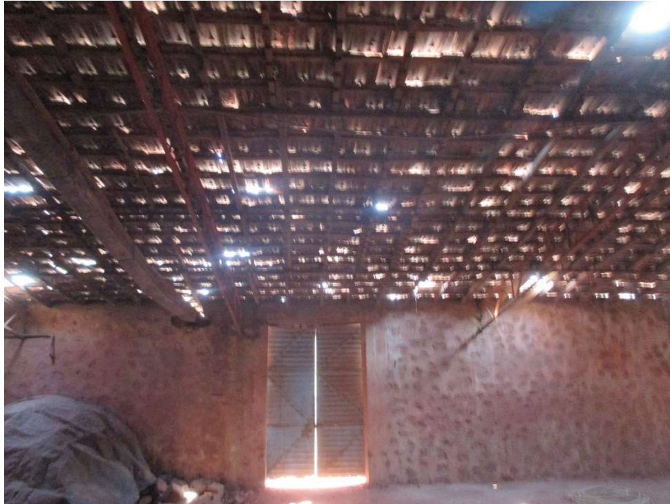
Figure 13: Potentially Thermally Advantageous Porosity of Mangalore Tile Roofing
