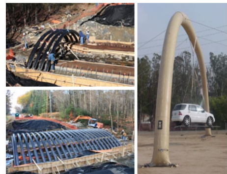
Figure 8. left: composite bridge arch right: airbeam.
