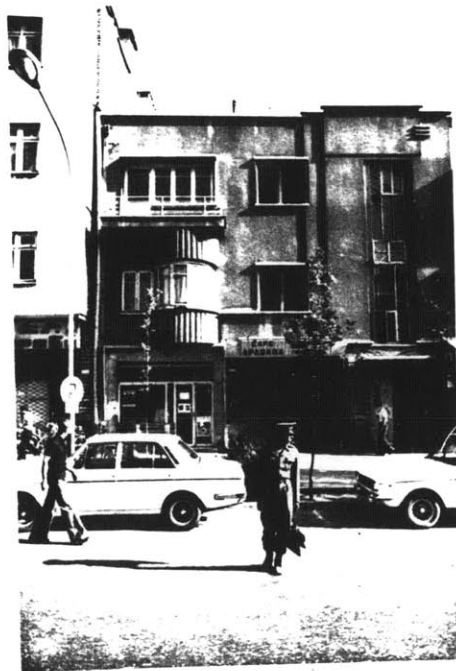
Fig. 3.63 Three story rowhouses along Shahreza Avenue
