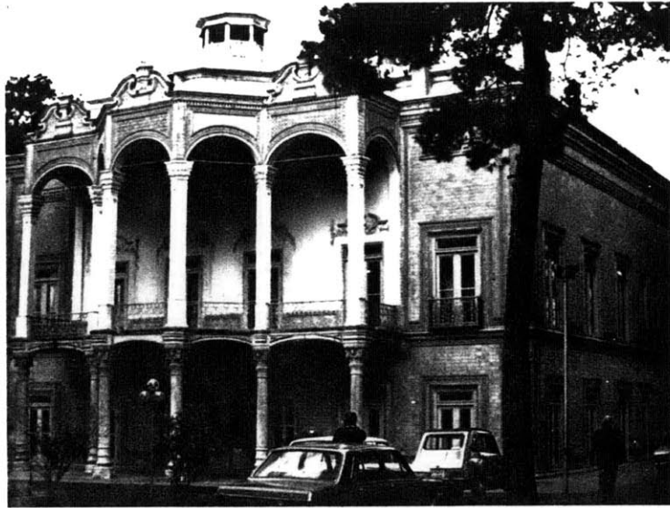
Fig. 3.27 Front facade and entry portico of Sardar Asad house
