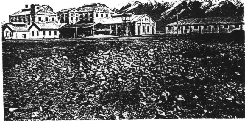
Fig. 2.120 Karaj sugar refinery, 1933-34
