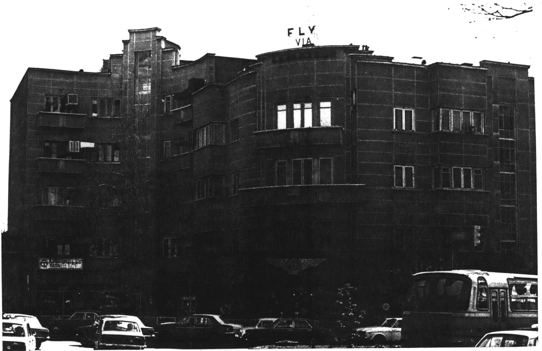
Fig. 2.22 Apartment building on Shahreza Avenue
