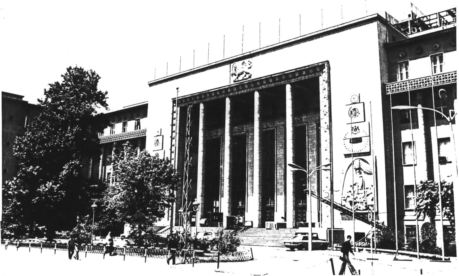
Fig. 2.89 Ministry of Justice, main facade
