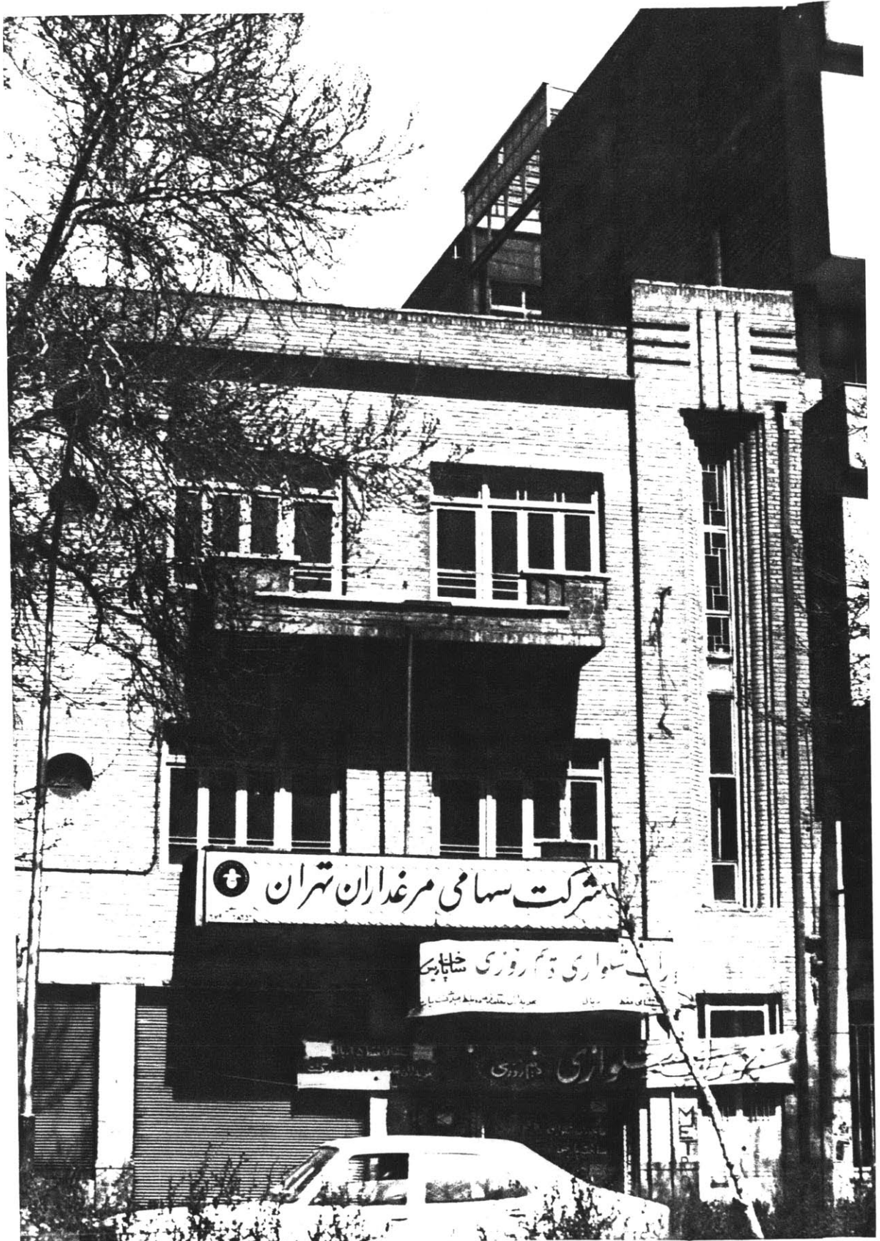
Fig. 3.52 Use of brick in residential architecture
