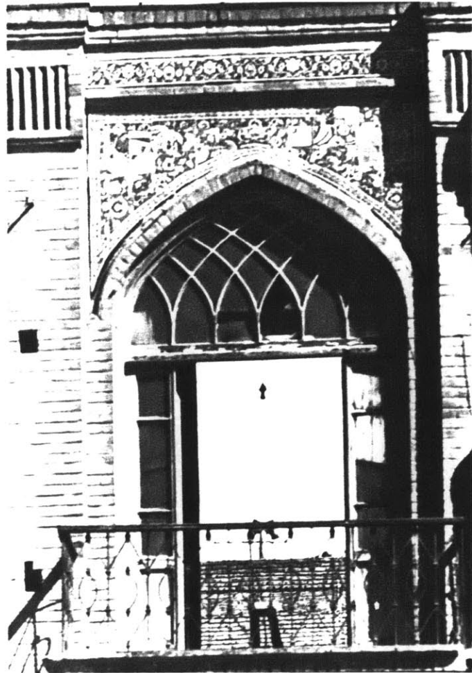
Fig. 3.61 Window details of rowhouses along Shahabad Street Note false facade
