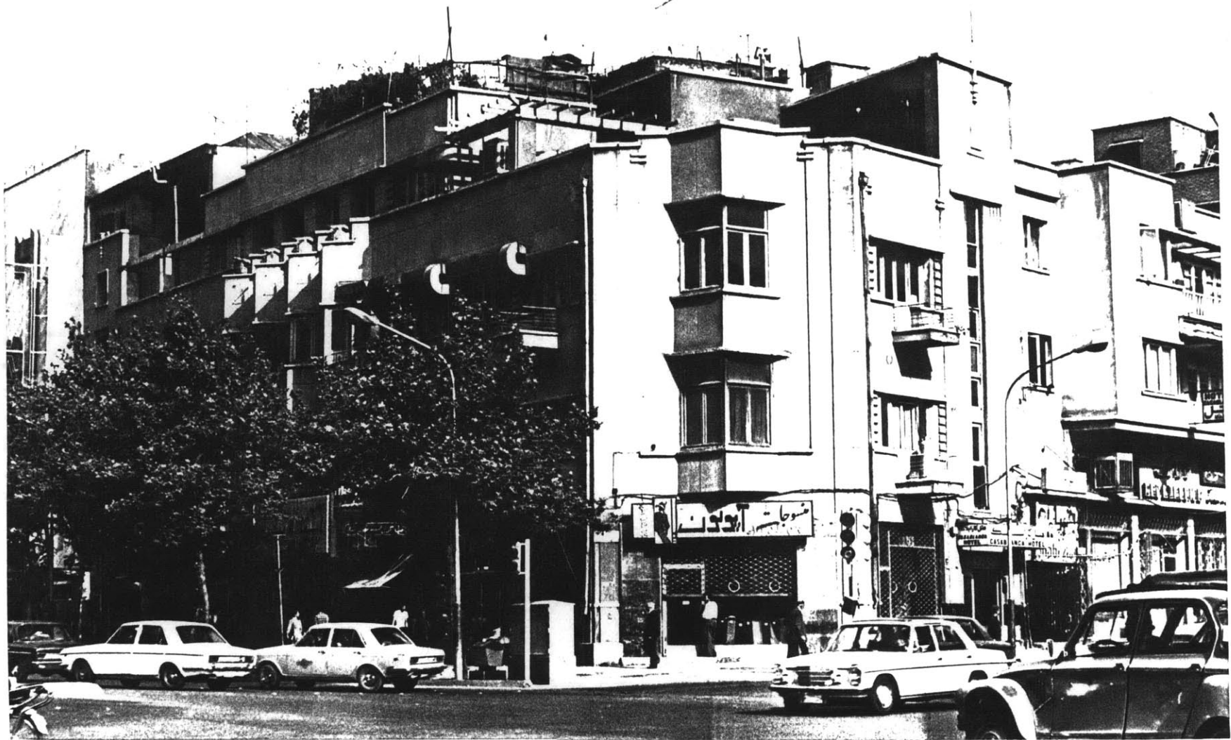
Fig. 2.21 Apartment building on Shahreza Avenue
