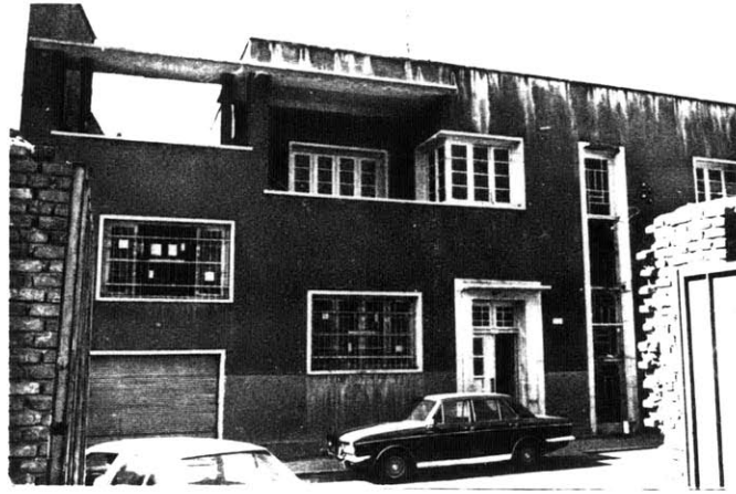
Fig. 3.67 Street elevation of rowhouse at 100 Moshtaq Street
