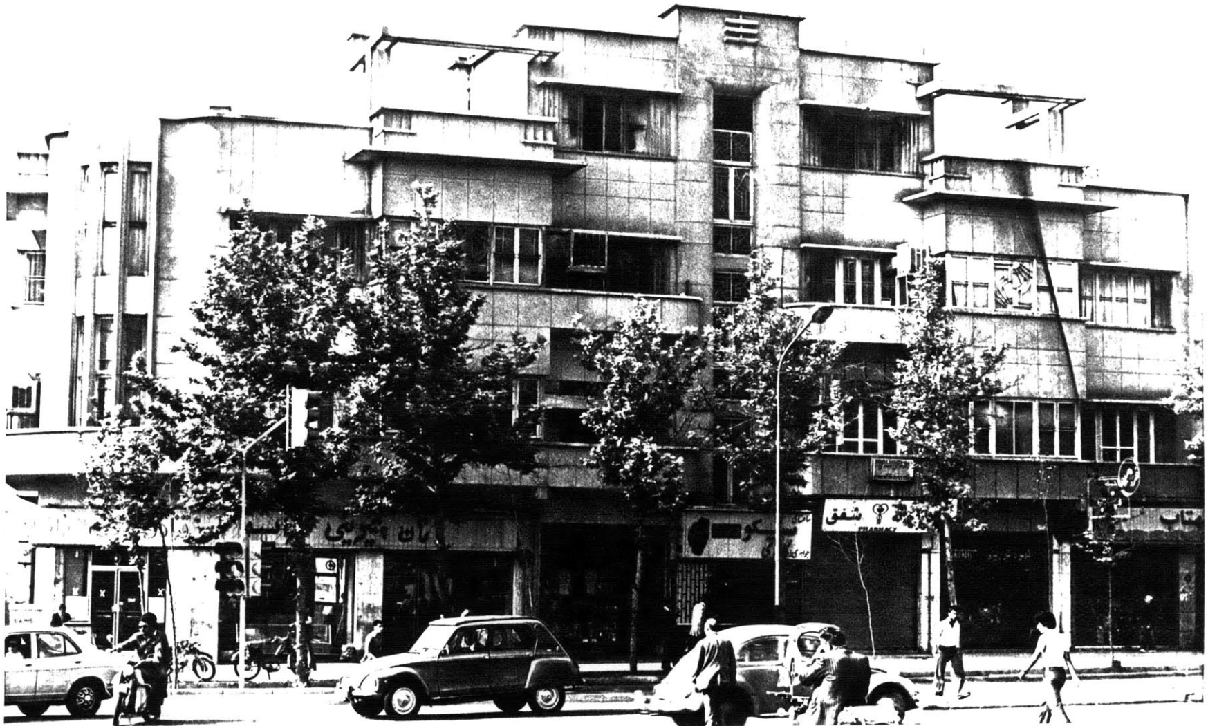
Fig. 3.93 Main elevation of apartment on Shahreza Avenue and Abu Reyhan Street
