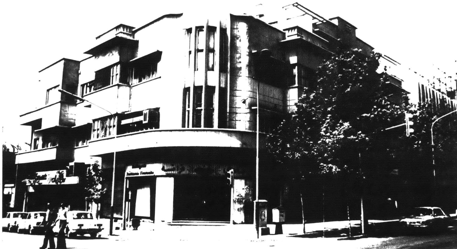
Fig. 3.95 Corner elevation of apartment on Shahreza Avenue and Abu Reyhan Street
