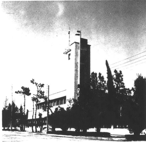
Fig. 2.149 Bank-e Melli, Hospital by Foroughi
