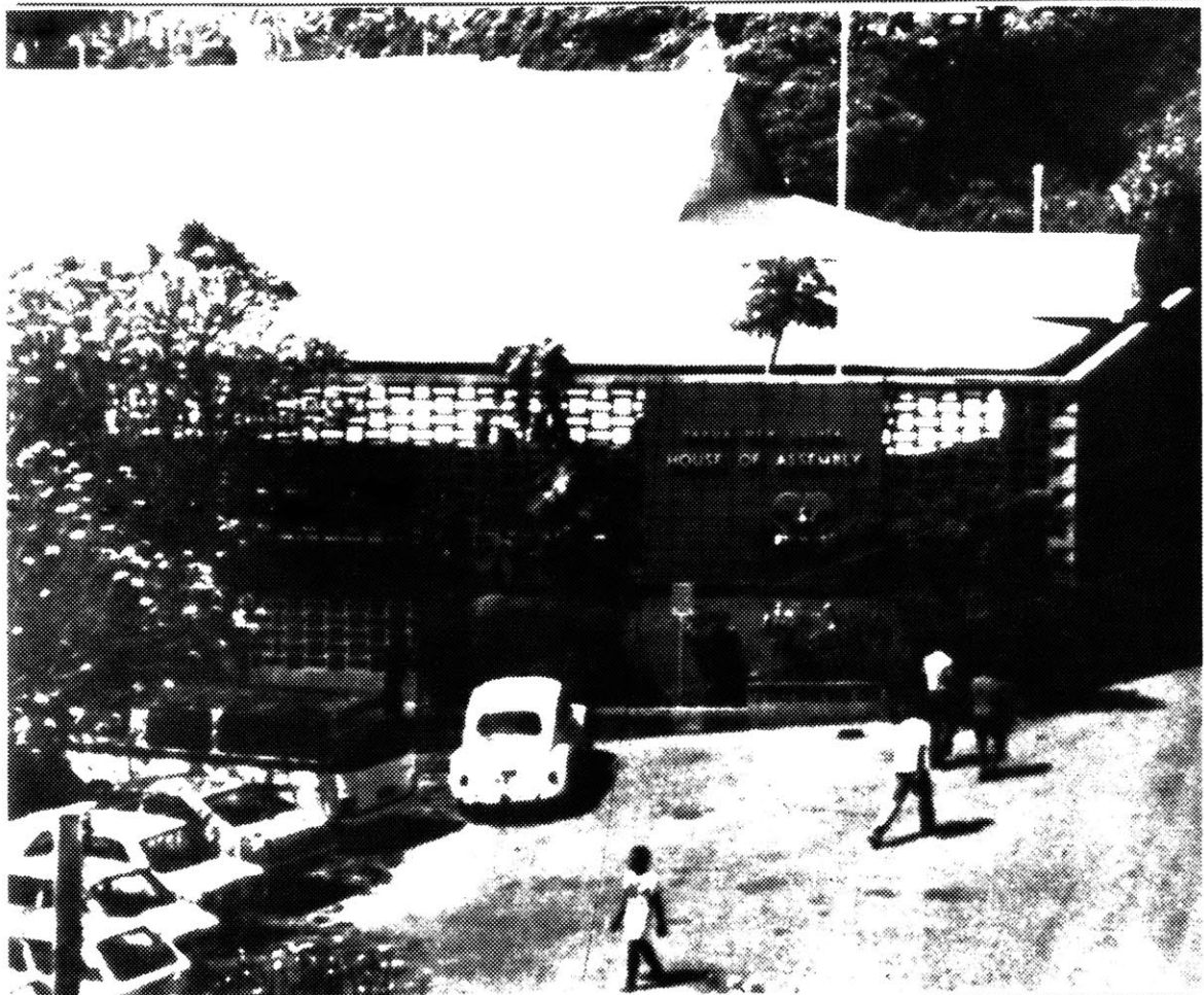
50. Old Assembly Building, Port Moresby
