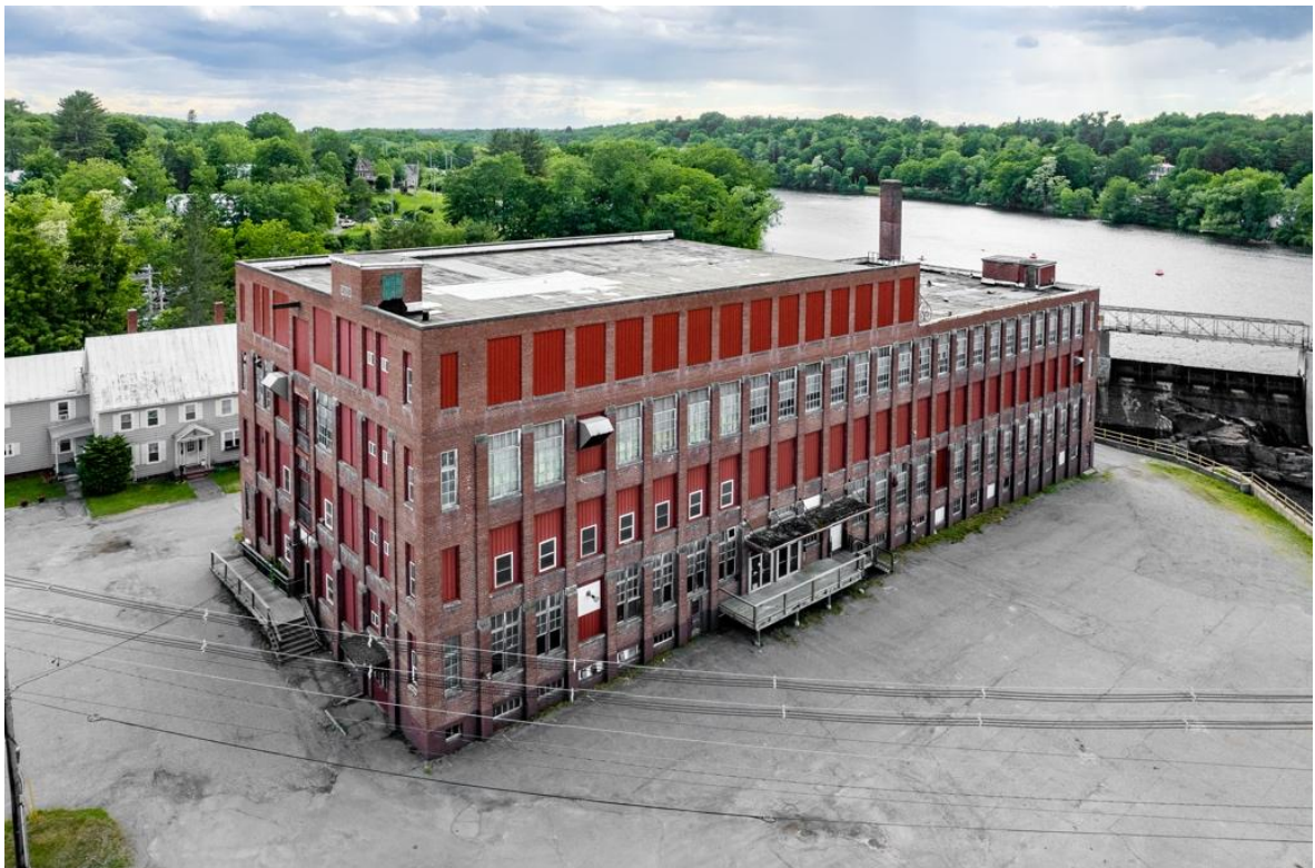
Figure 5.1: Current condition of 7 Island Avenue, Skowhegan Maine. Photo May 2022
