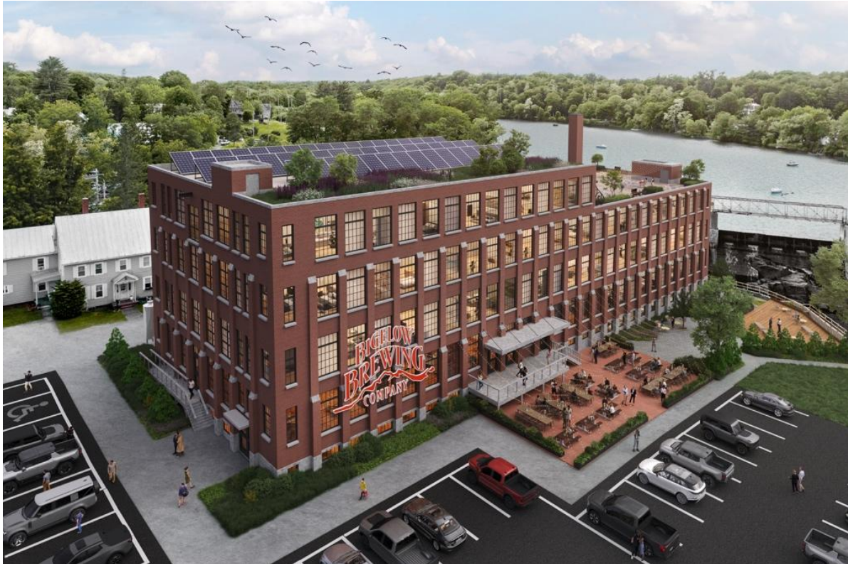
Figure 5.2: Computer generated 3D rendering of 7 Island Avenue, Skowhegan Maine, 04976 intended to be complete in Fall 2024
