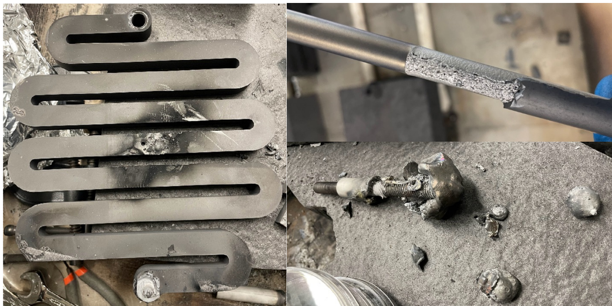
Figure 20 – Arc-melted tungsten leads and damaged graphite heater due to arcing during high-temperature operation.
