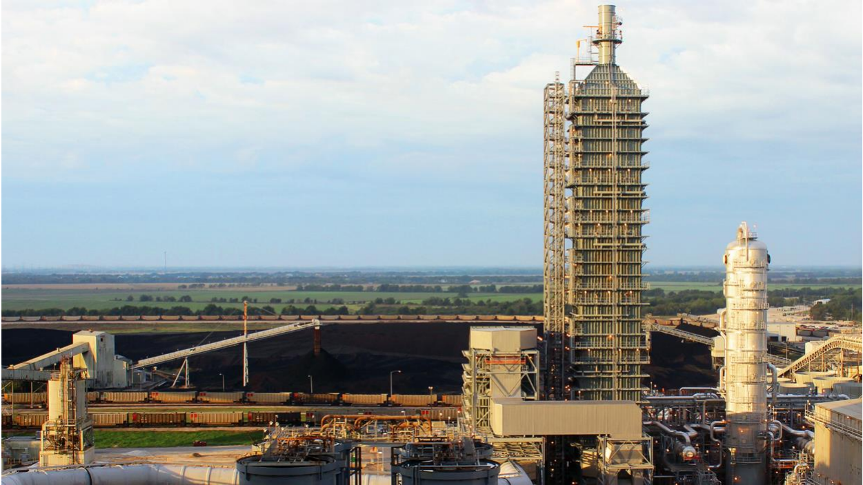
Figure 5-2. Absorption tower at Petra Nova CO 2 capture facility, Texas. This is one of the world's largest carbon capture and storage facility that costed more than $0.5 billion to construct. The absorption tower is more that 380 ft tall. 176 : Global CCS Institute.
