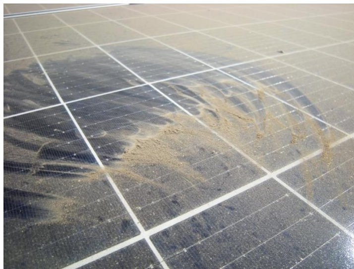
Figure 1-1. Dust accumulation on solar panels. Blocking of sunlight and the resultant loss of power output due to dust accumulation on solar panels is by far the biggest operational challenge
