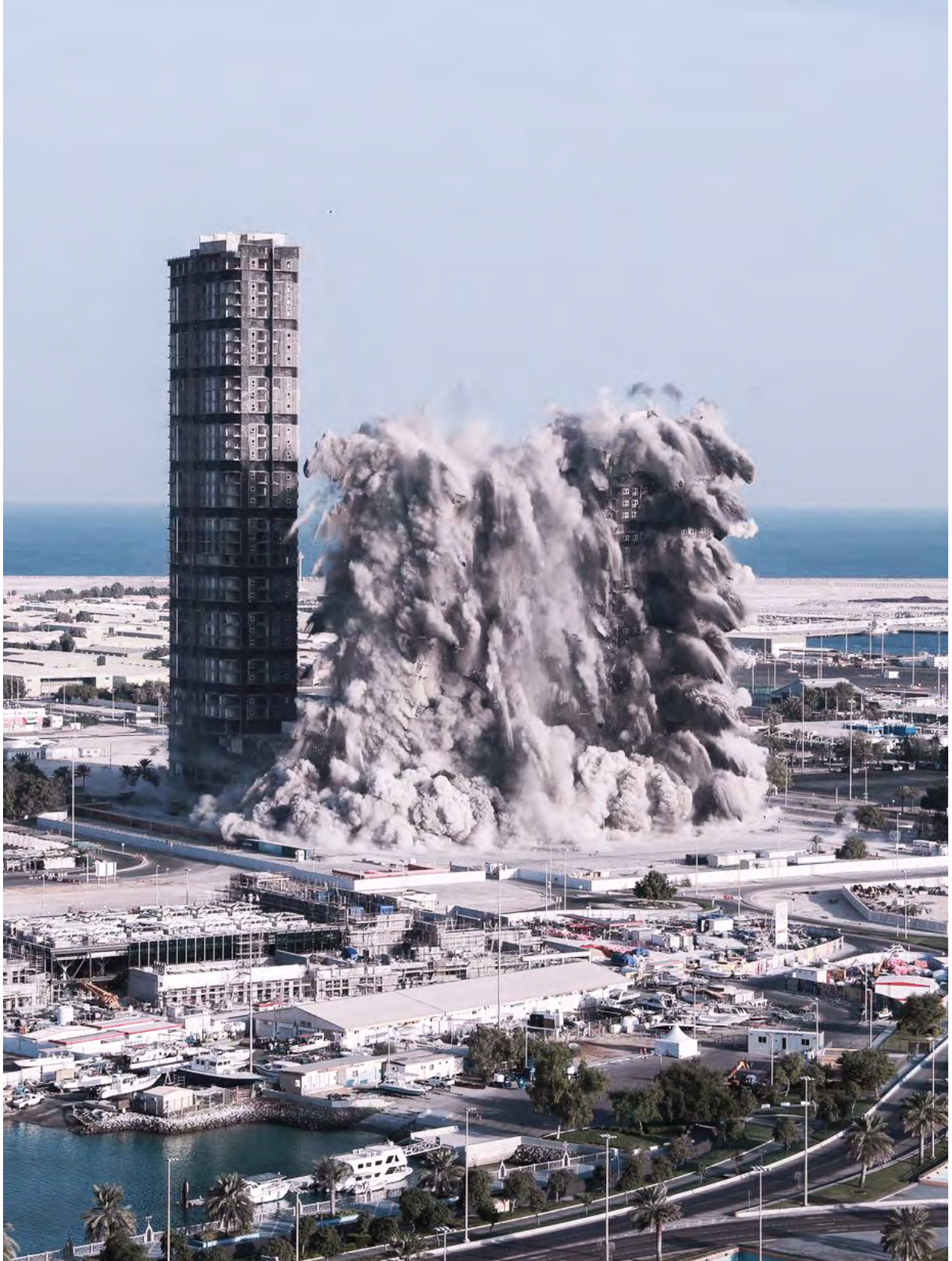
Fig 17. Demolition of Mina Plaza Towers
