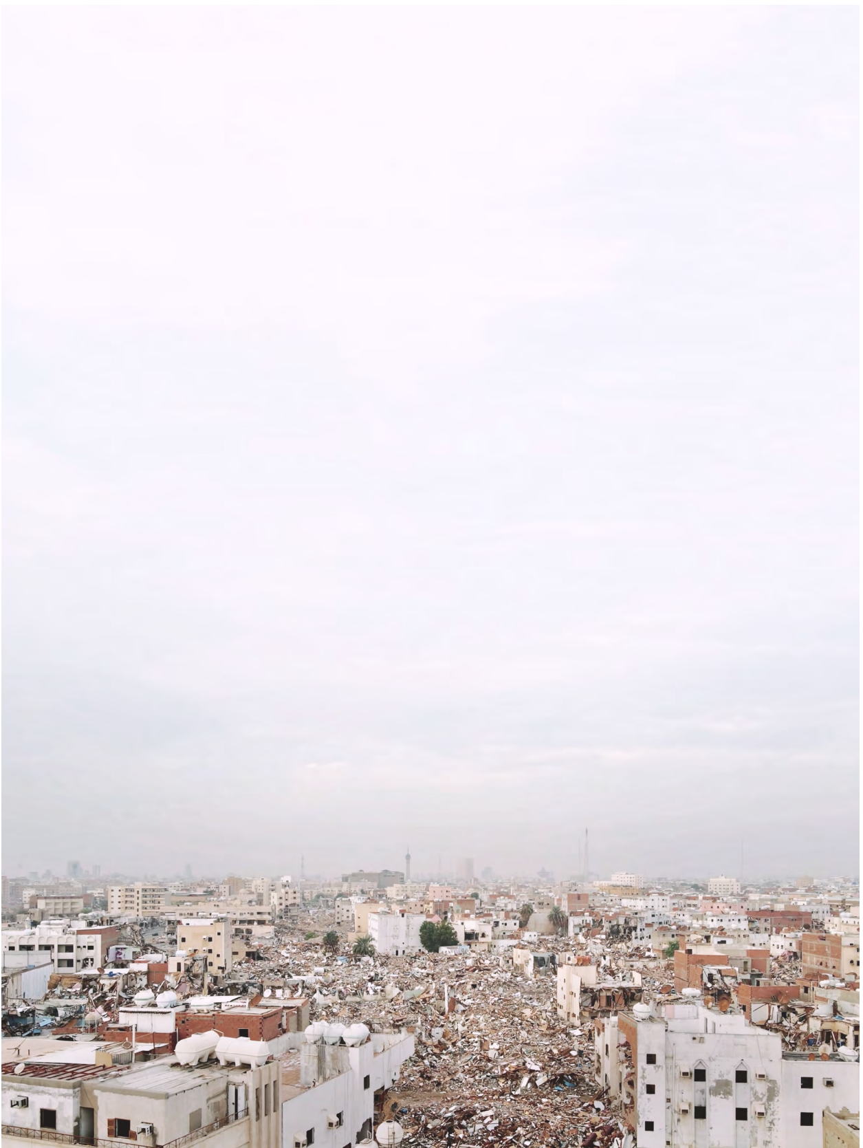
Fig 14. Demolition of the city of Jeddah.
