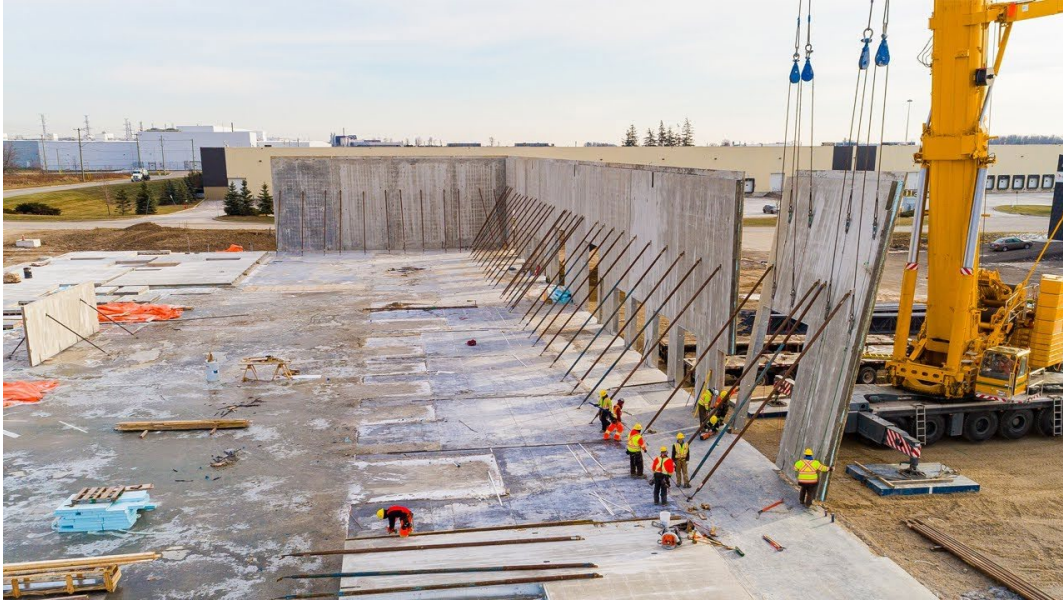
Figure 10 - Tilt-Up Construction (Tilt-wall Ontario Inc., 2022)
