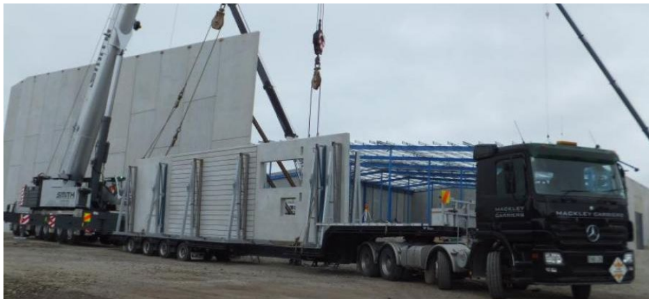
Figure 12 - Pre-Cast Panel Transportation (Mackley Carriers, n.d.)
