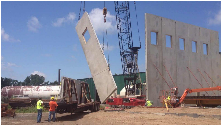
Figure 11 - Pre-Cast Panels Installation (Precast Concrete Wall Panels, n.d.)
