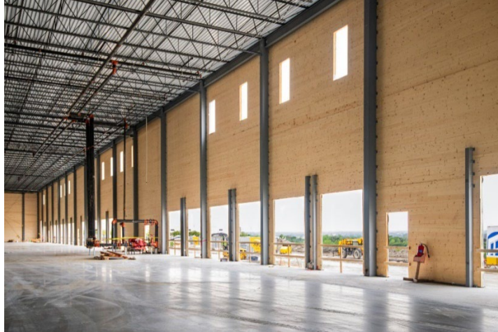
Figure 18 - Interior view - USAA CLT Warehouse (Frank, 2023)
