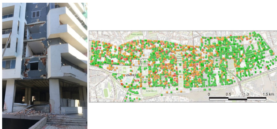
Fig. 2 a Damage and collapse of infill walls in a 2-storey RC building in Durrës during Albania earthquake (MW 6.4) of November 26, 2019 [18] and b building usability in the Lower town of Zagreb after the M_w 5.4 Zagreb (Croatia) earthquake of March 22, 2020 [1]
