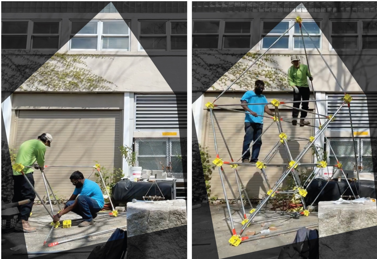
Figure 4-5: Sequence of build one. Following the concept model, the assembly order is based on human intuition. Time to assemble is under two hours.
