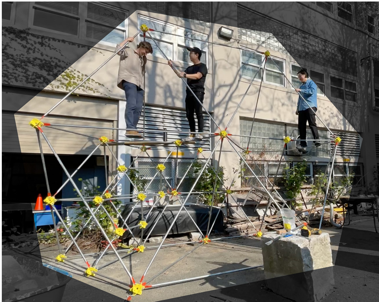
Figure 4-6: Build two. The structure is extended by removing nodes from overly stiff sections and reusing them elsewhere. Multiple individuals contribute to the assembly.
