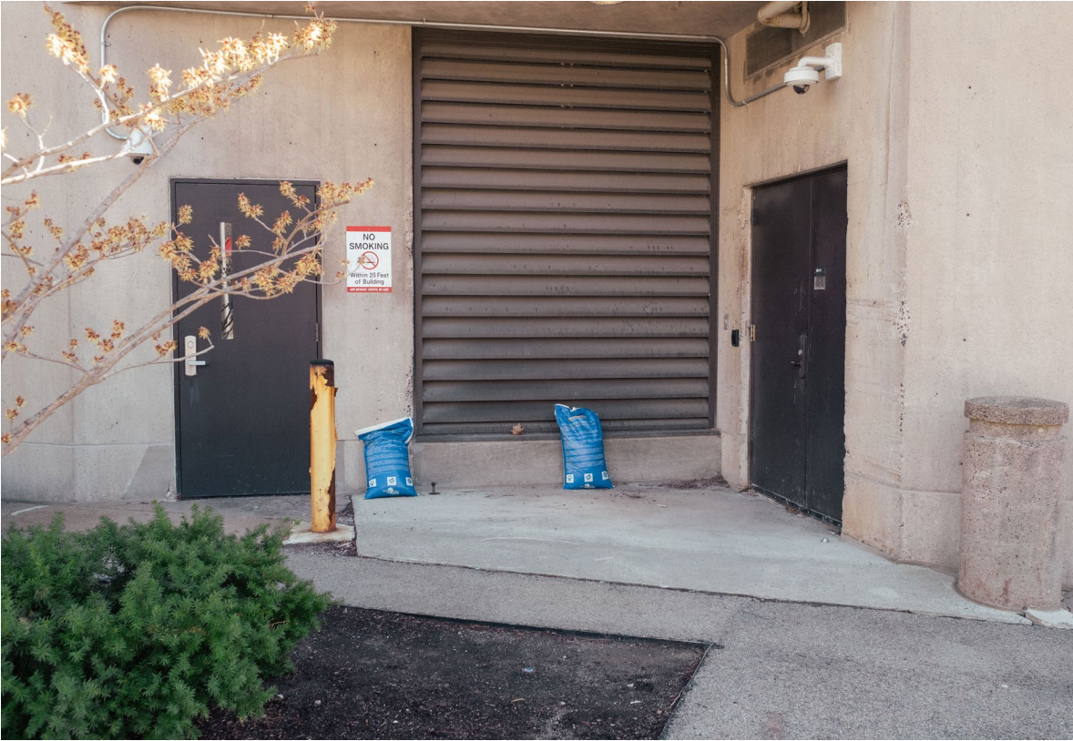
Figure 28 Photograph of secondary entrance to building 66.
