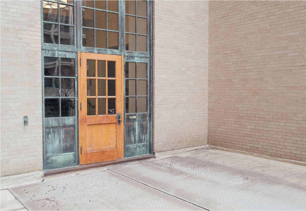
Figure 29 Photograph of an entrance (locked) to building 3.
