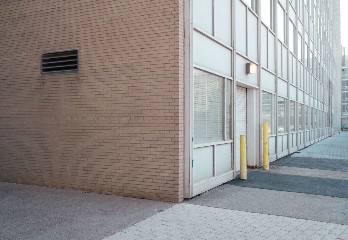
Figure 26 Photograph of the corner of building 56.
