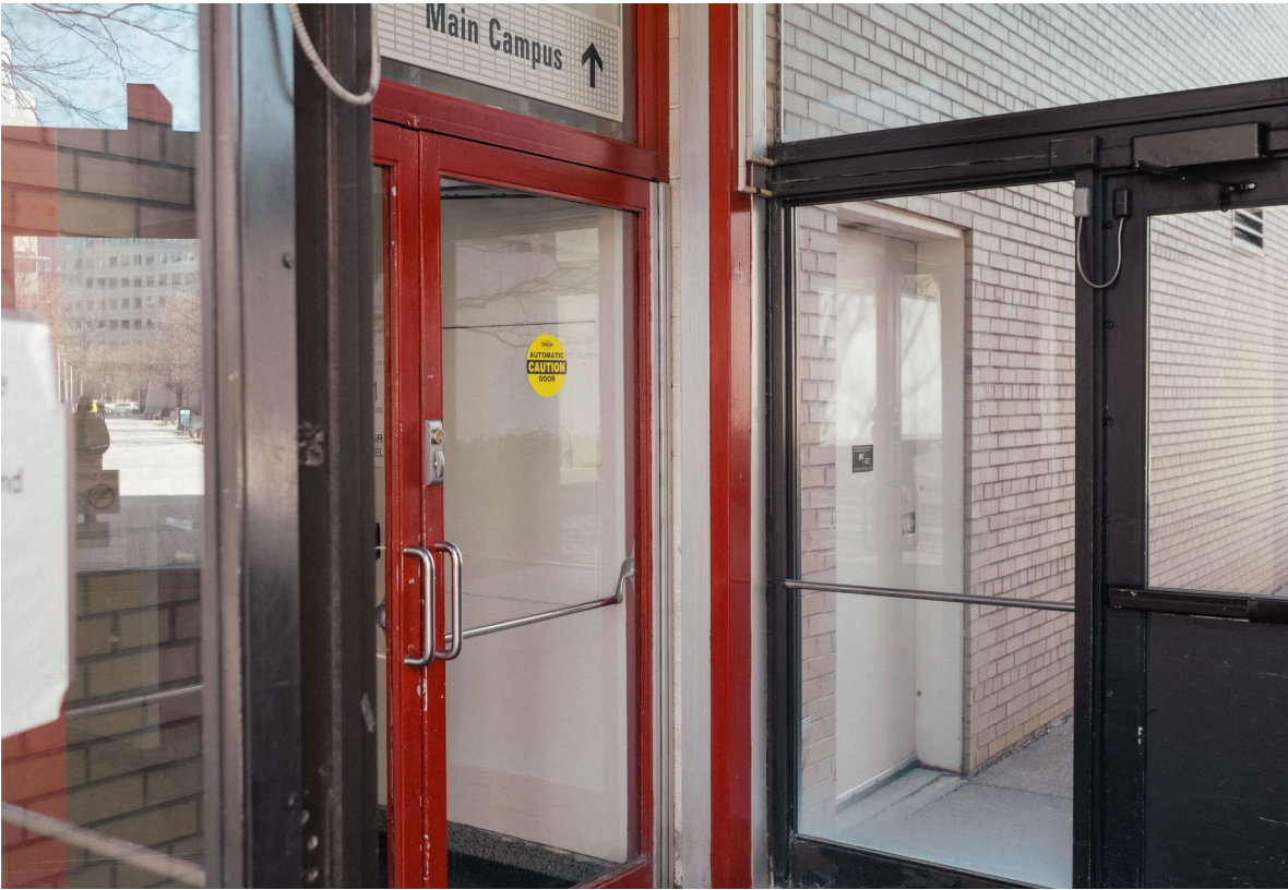
Figure 27 Photograph of the triple entrance zone from building 56 to building 66.
