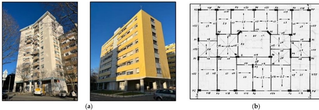
Figure 4.5: Photos from 1961-1980 Typical Reinforced Concrete Buildings and Floor Plans in Lisbon (Xavier et al., 2022).
