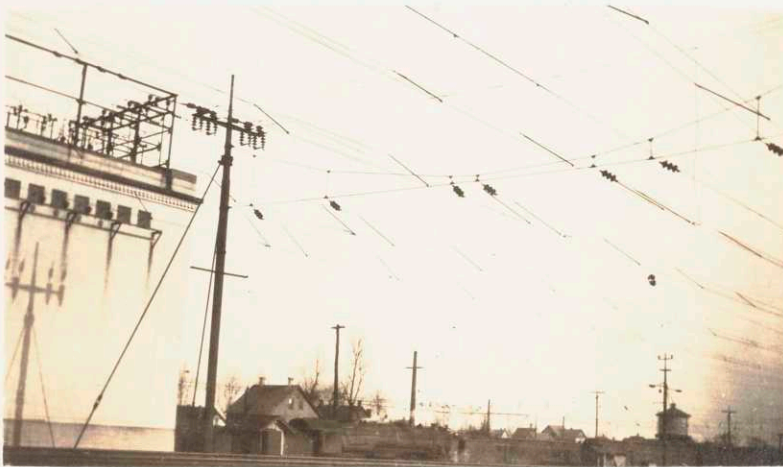
Sub-Station No. 4 - Paoli Paoli Yards in the Background
