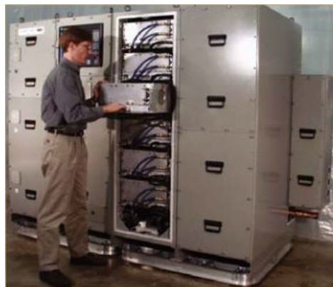
Figure 3-3: SATCON PCM-1 Conversion Sections [4]
