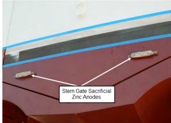
Figure 1-4: New Stern-gate Zinc Anodes
