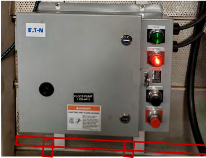
(a) White welded brackets installed on outboard bulkhead stiffeners. Bracketry locations shown in red.
