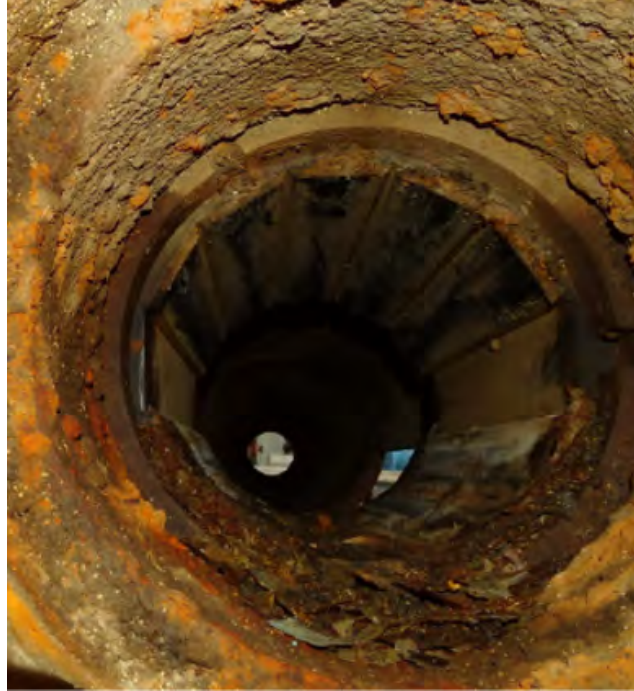
Figure 1-2: FRC Bearing Housing immediately after dry docking
