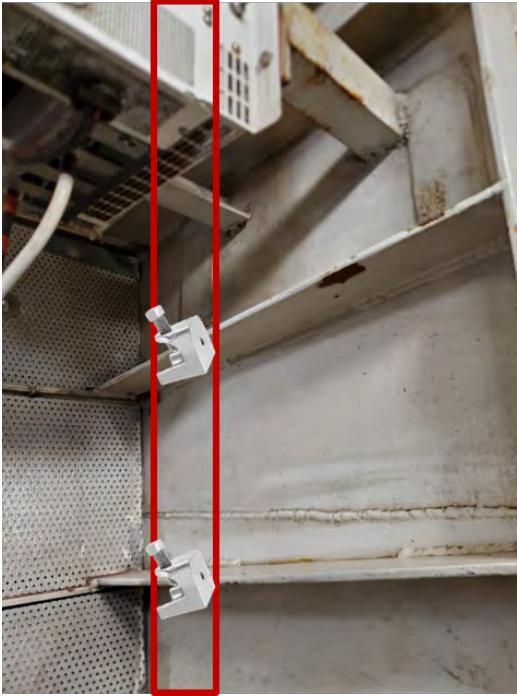
(a) Location to mount Unistrut on aft bulkhead. Unistrut will extend down from permanently mounted “L” brackets to provide anchor points for other bracketry. It will also bolt to beam clamps on horizontal stiffeners.
