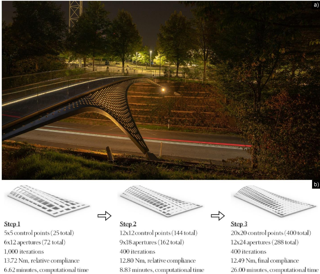
Figure 5-3: Examples of work expanding the fields of structural patterning of shell structures a) Footbridge TRUMPF in Ditzingen, Germany (2018), b) adaptive framework to reduce computational time in the design process of perforated shell structures (Rivera et al., 2020)
