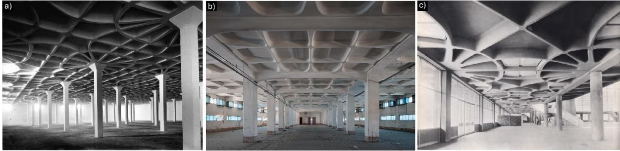
Figure 2-7: Images of Pier Luigi Nervi's famous floor concrete ribbed floor systems, a) Gatti Wool Factory, Rome 1953, b) Tobacco Factory, Bologna 1952, c) The Palace of Labor, Turin 1959
