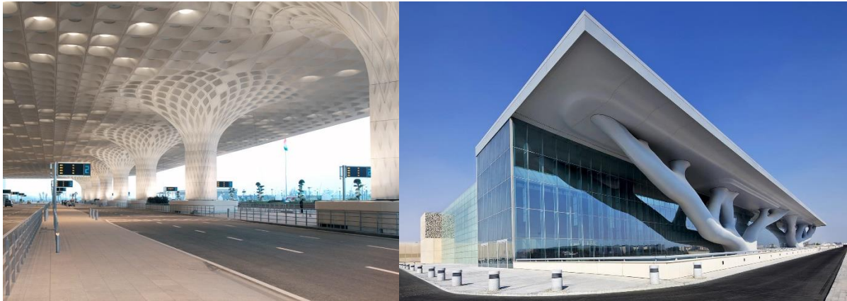
Figure 5-4: Images of systems evoking structural logic and expression but realized via conventional systems and cladding. Left: Chhatrapati Shivaji International Airport, Right: Qatar National Convention Center
