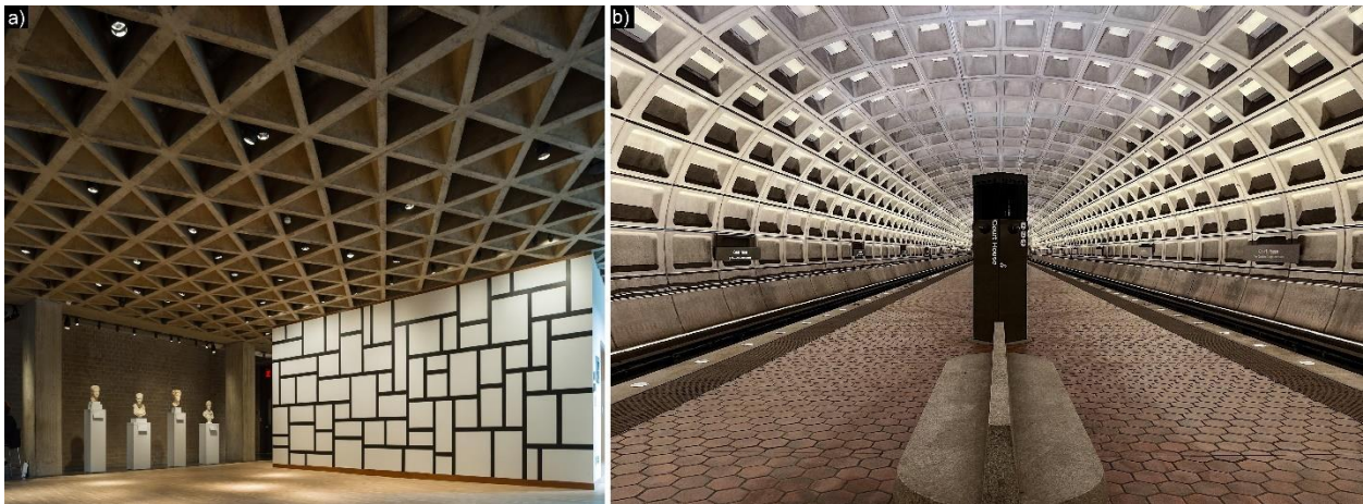
Figure 2-8: Renown built examples in the United States of waffle slabs, a key spanning system in many brutalist structures. Examples featured include a) The Yale University Art Gallery and b) Washington D.C. Metro Train Stations
