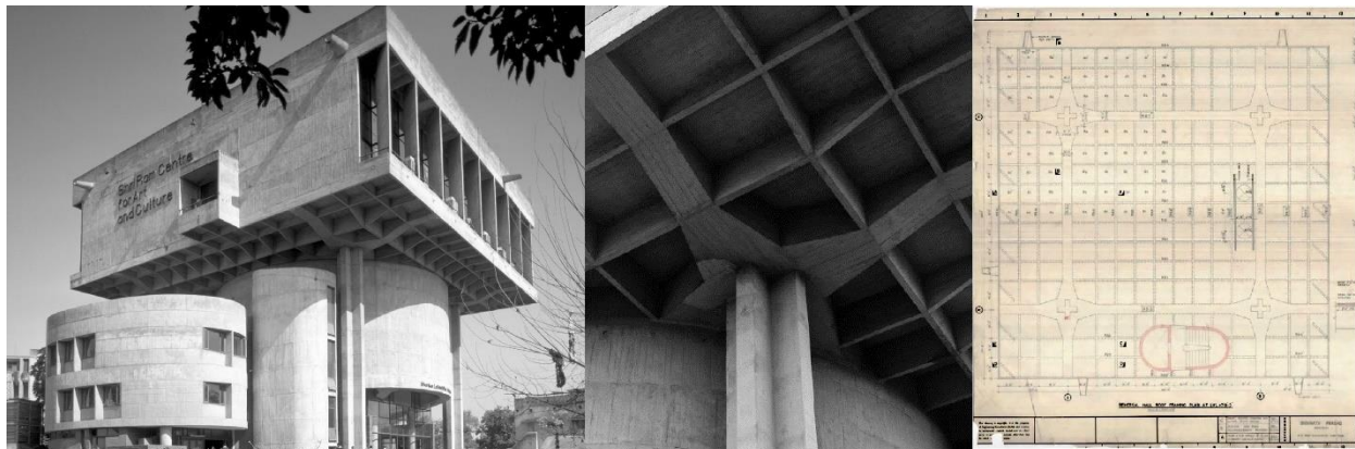
Figure 5-7: Left - ShriRam Centre for Arts and Culture, New Delhi, India, middle – close up shop of shaped waffle slab ribs for cantilevered roof element and right – roof framing drawing.
