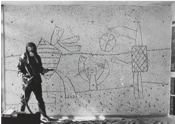
Figure 5.4.3. Sandblasted mural: Carl Nesjar sandblasting Picasso's The Beach onto the walls of Høyblokka - Reprinted from kunstkritikk.com , 1959.
