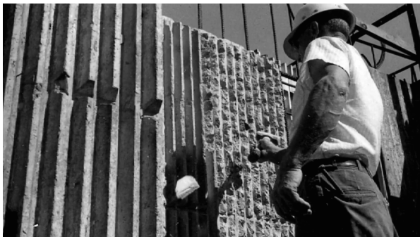
Figure 5.4.1. Crafting surface: Construction worker hammering façade of Yale art and architecture building designed by Paul Rudolph - Reprinted from dirtymodernscoundrel.blogspot.com , 1963.
