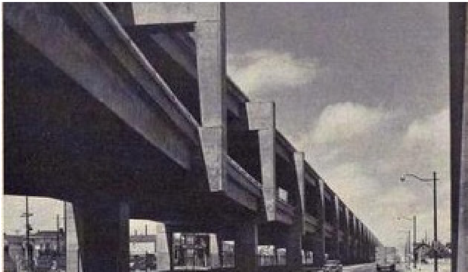
Figure 25: The double-decker Cypress Freeway (California Highway and Public Works)
