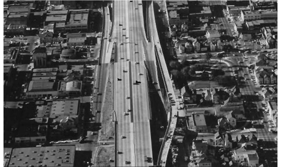
Figure 24: Cypress Freeway ramps (Remembering 7th Street)
