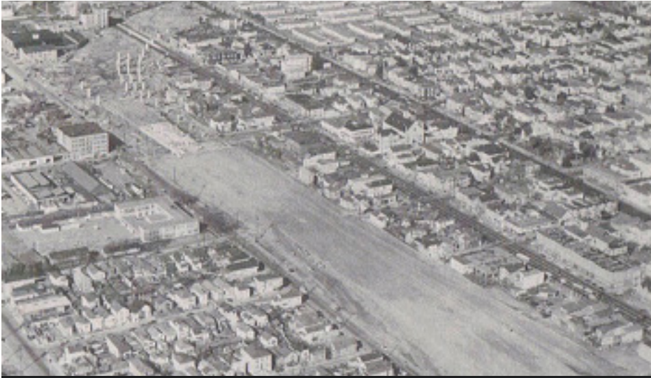
Figure 23: Land cleared to build Cypress Freeway (Oakland Tribune Collection)
