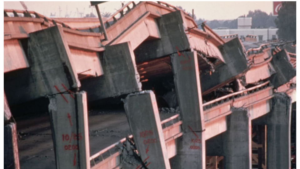
Figure 26: Cypress Freeway collapse during the 1989 Loma Prieta Earthquake (Jim Sugar/Corbis Historical)
