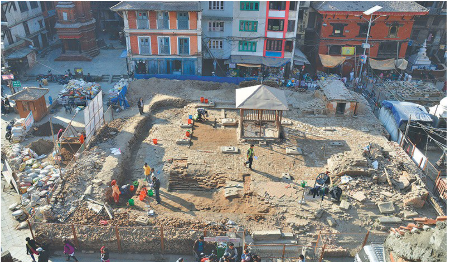
Figure 1: Kasthamandap Reconstruction Site | Anie Joshi
