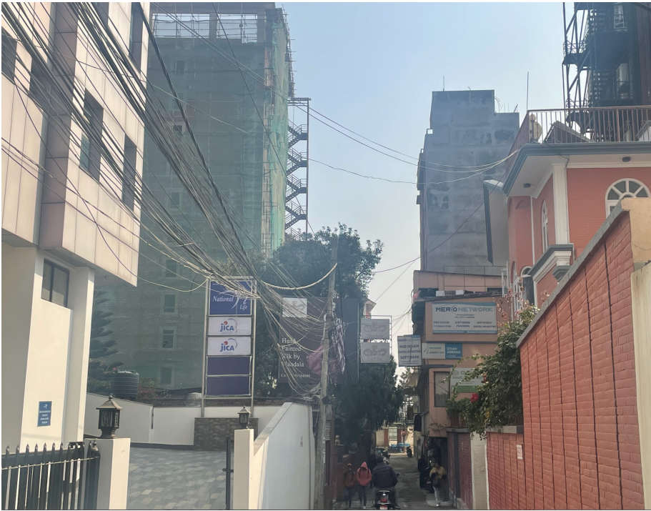
Figure 19: JICA headquarters in Ward no.2, Kathmandu
