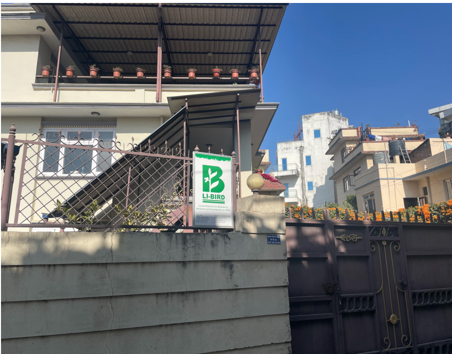
Figure 18: Residential quarters for Li-Bird in Ward no.2, Lalitpur
