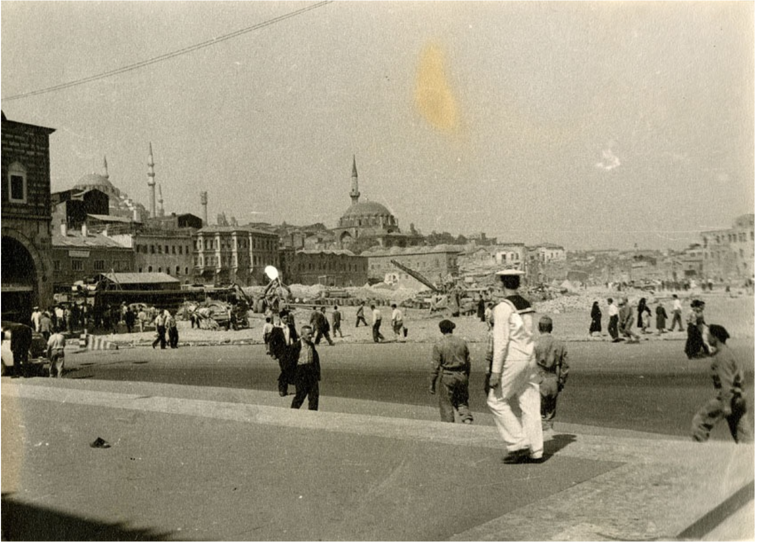
Figure 35 – View of Eminönü Square site being demolished, undated photograph, from Académie d'architecture, Cité de l'Architecture et du Patrimoine, Archives d'architecture du XXe siècle, Fonds Henri Prost, 343 AA 67/1.
