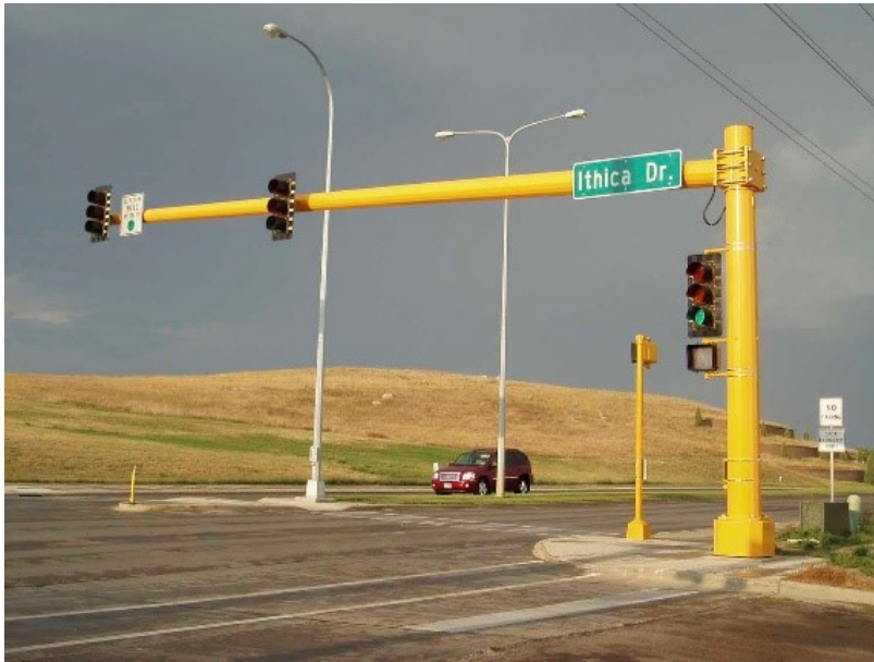
Figure 2-9: Cantilevered beam to support traffic lights
