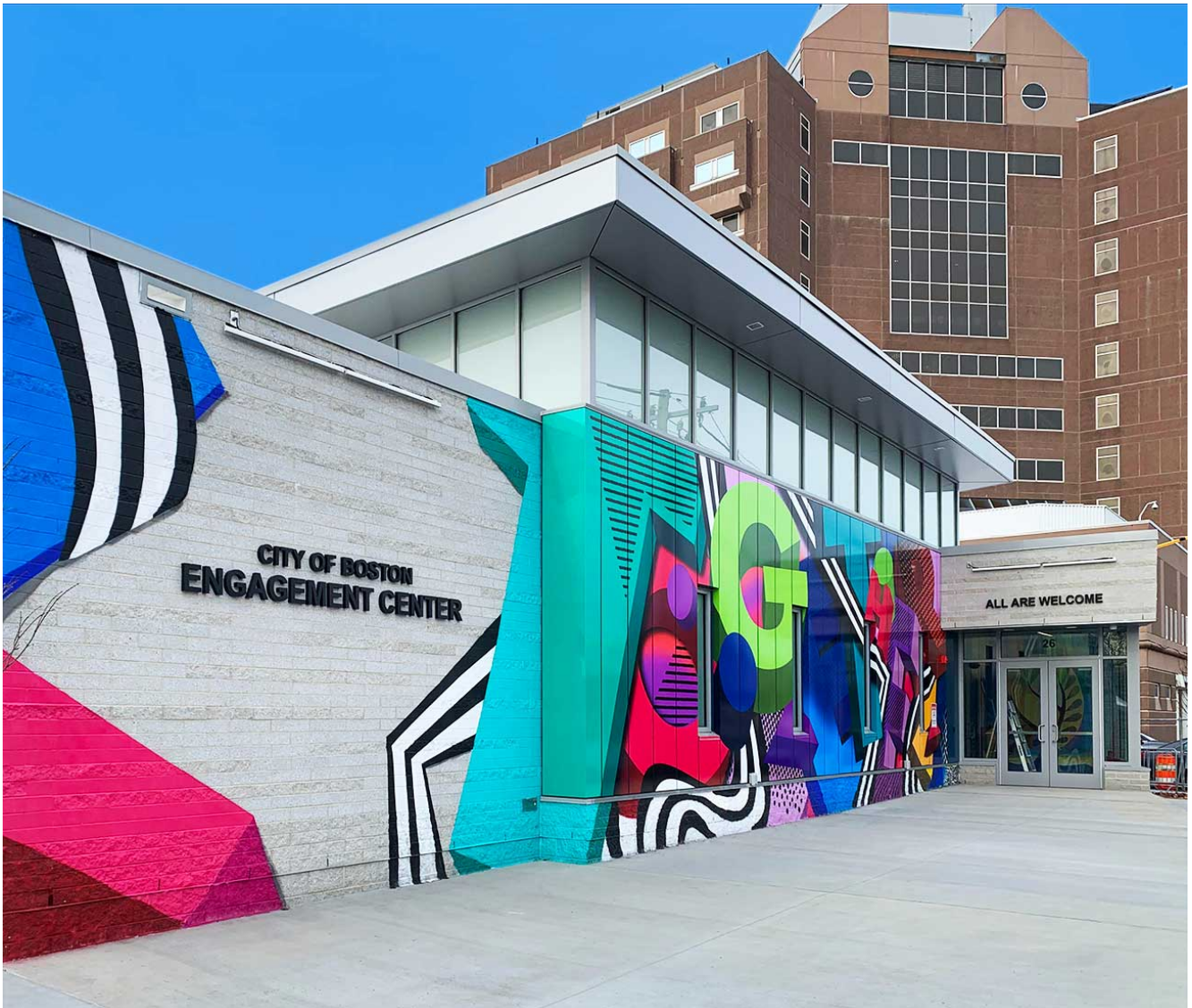
Outside the new Engagement Center, with an “ALL ARE WELCOME” sign and mural by artist Mz.Icar. The South Bay Jail sits in the background. / Christian Phillips Photography for saam architecture, 2021.
