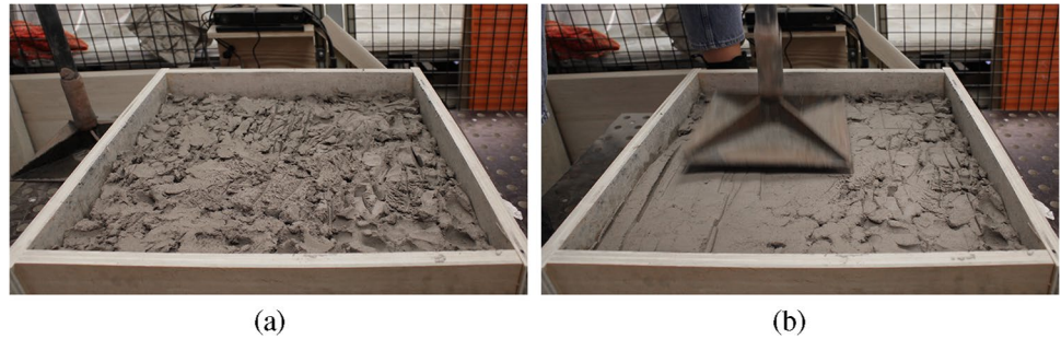
Fig. 16 (a) Filling timber formwork with adobe mixture, and (b) tamping adobe
