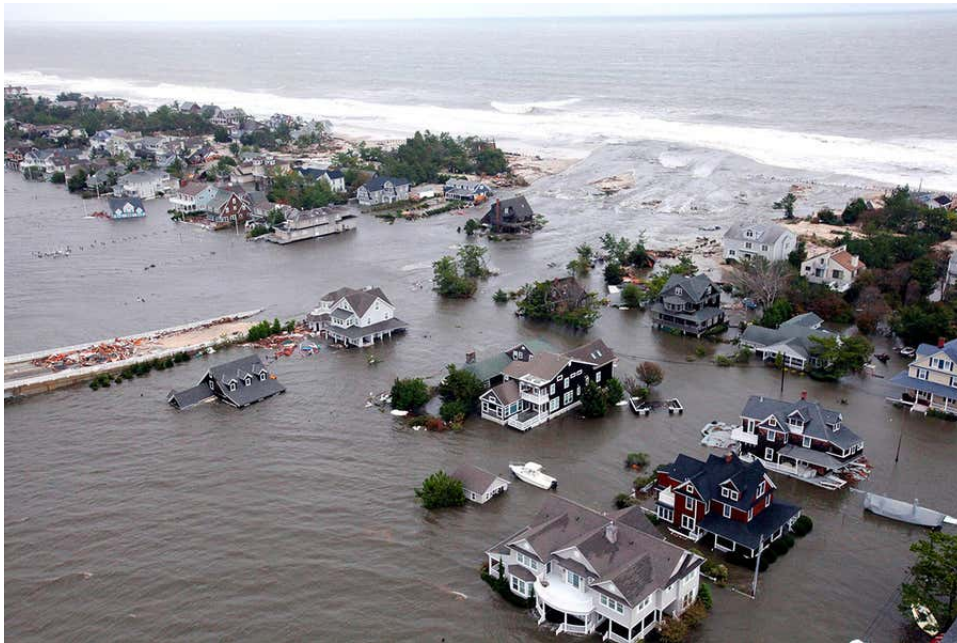
Figure 3-8: Storm surge flooded the base of the Mantaloking Bridge and State Route 35 in Mantaloking, New Jersey, such that an inlet formed between the Barnegat Bay and Atlantic Ocean. Photograph courtesy of Master Sergeant Mark Olsen of the United States Air Force.
