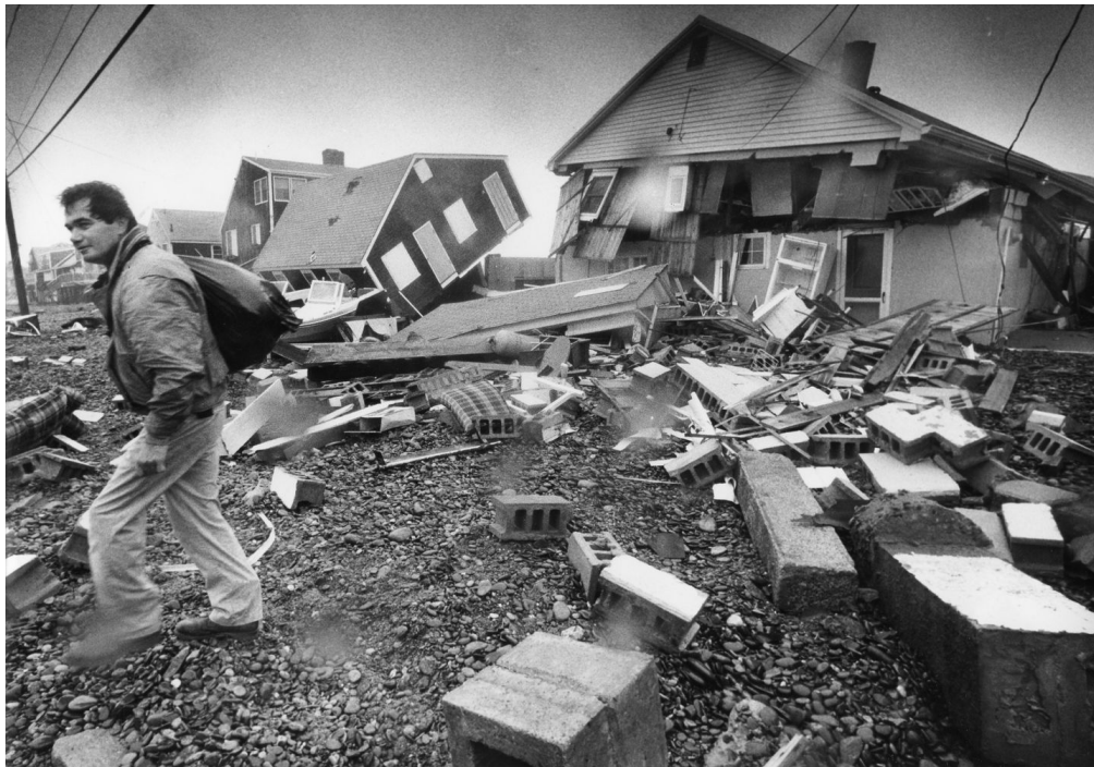
Figure 3-4: Destruction caused by the wind field of the Perfect Storm in Scituate, Massachusetts. Photograph courtesy of Barry Chin of the Boston Globe.
