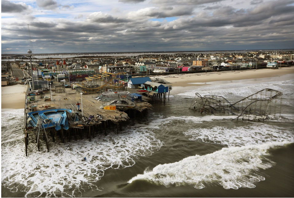
Figure 3-7: The Casino Pier amusement park in Seaside Heights, New Jersey, destroyed by Superstorm Sandy. The Jet Star roller coaster is seen partially submerged in the surf zone, where it would remain until May. Photograph courtesy of Mario Tama of Getty Images.
