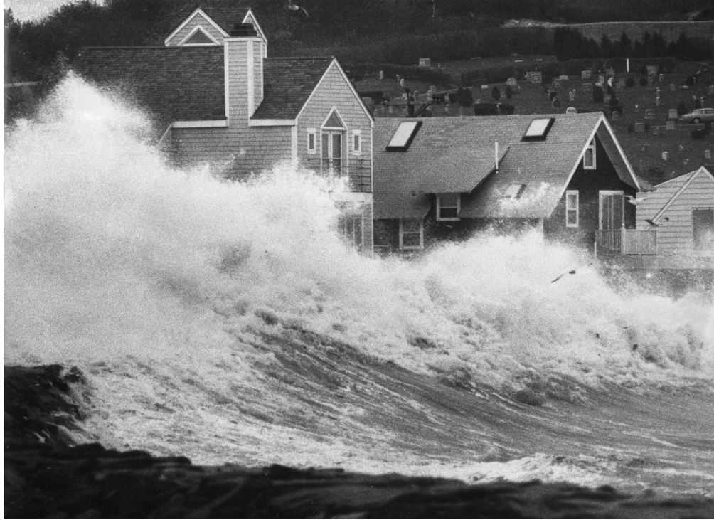
Figure 3-3: Waves crashing into homes Scituate, Massachusetts, due to the passage of the Perfect Storm. Photograph courtesy of the Boston Globe Staff.
