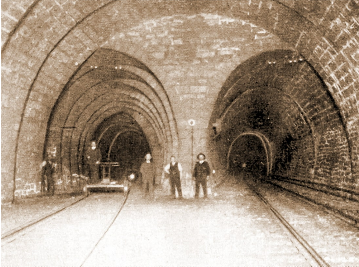
Figure 2-7: Simplon tunnel construction, 1900s [Wonders, 2010].
