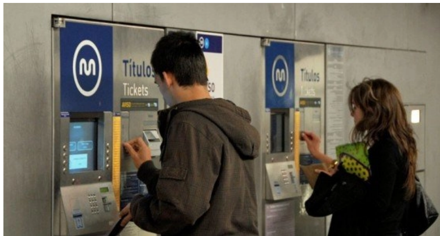
Figure 2-28: Andante Ticketing stations in a Porto Metro station [Guedes, 2017].
