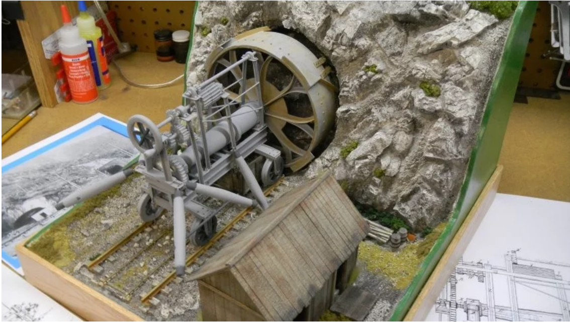
Figure 2-17: Model of Wilson Patent Stone Cutting Machine model used in the Hoosac Tunnel construction [Kelley, 2017].
