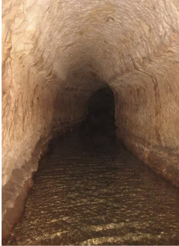
Figure 2-14: Gadhara Aqueduct in Jordan, 90-210 A.D. [Pafnutius, 2023].
