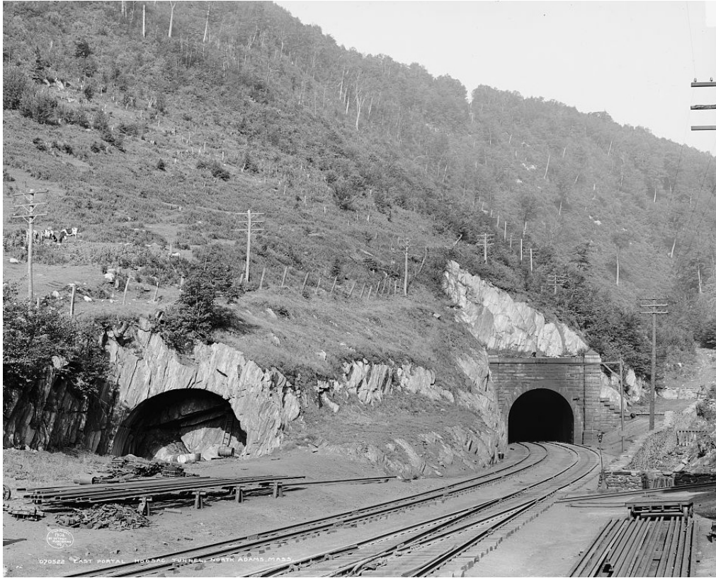
Figure 2-4: Hoosac Tunnel, Massachusetts, 1908 [Burns, 2022].
