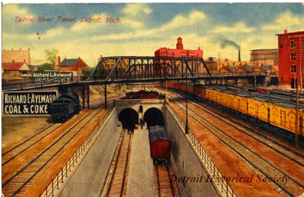
Figure 2-11: Michigan Central Railway Tunnel (also known as Detroit River Tunnel), 1910. [Gleit, 2016].
