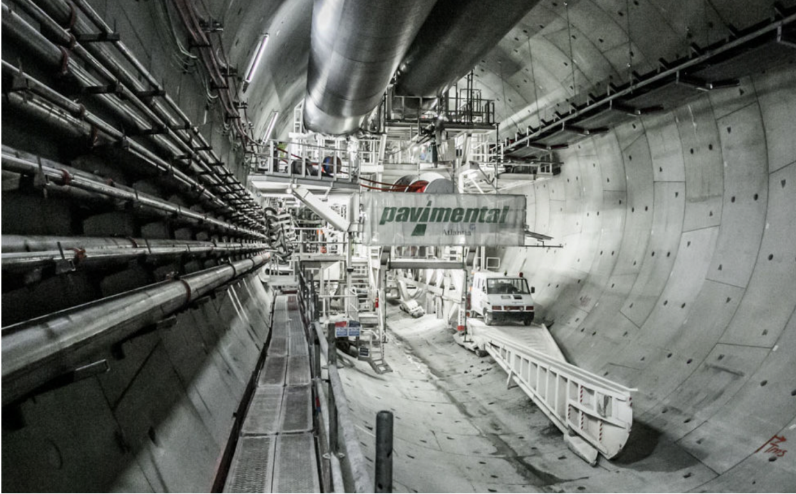
Figure 2-15: Saint Lucia tunnel between Bologna and Florence, 2020 [Formiche, 2020].
