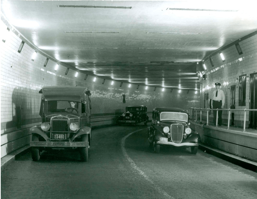
Figure 2-10: Holland Tunnel in 1928 [The Port Authority, 2016].
