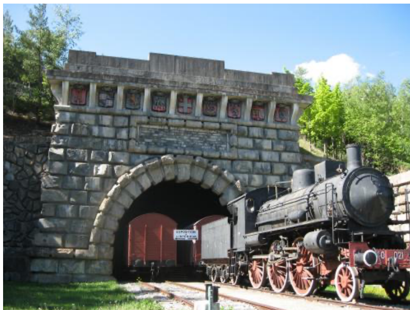
Figure 2-5: Mont Cenis tunnel, France [Cottet Dumoulin and Schueler, 2020].
