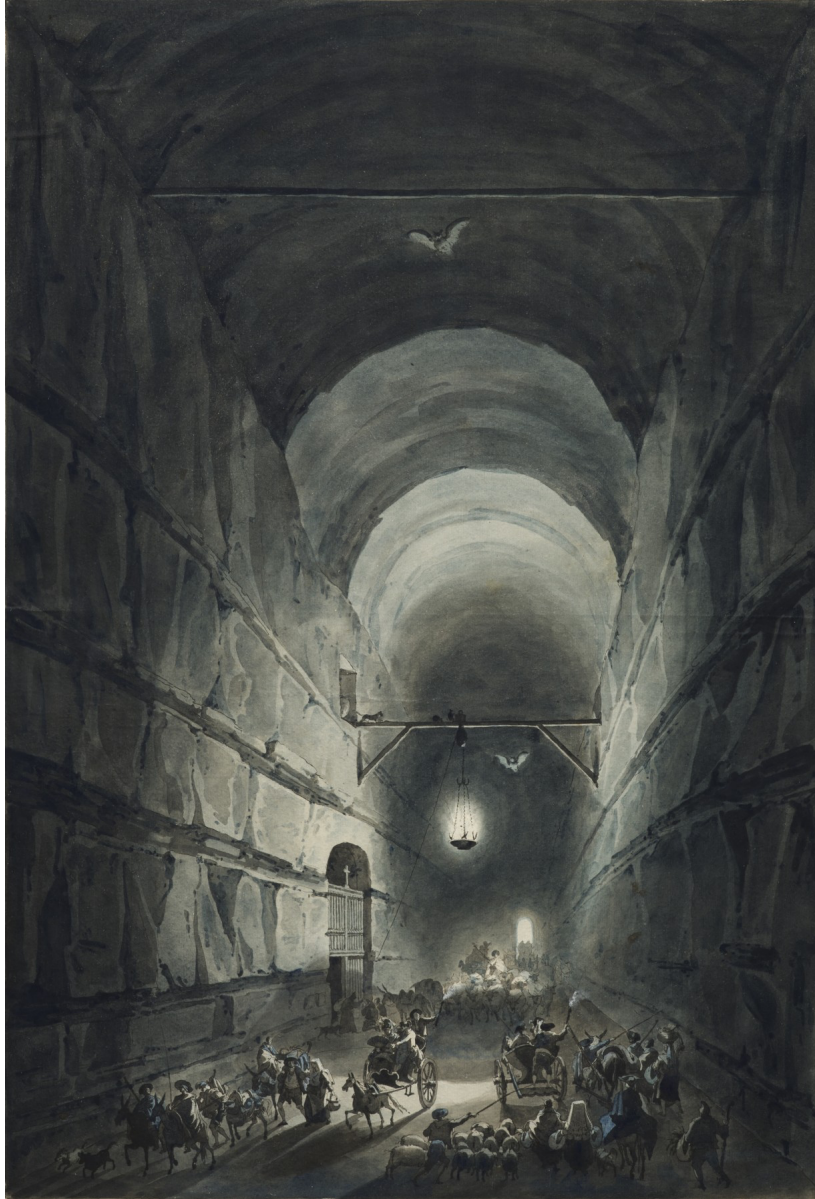
Figure 2-1: Pausilippo tunnel as depicted by Louis-Jean Desprez (1781-1784). The tunnel, built by the Romans was 4,800-foot-long, 25-foot-wide and 30-foot-high [Renard, 2020].
