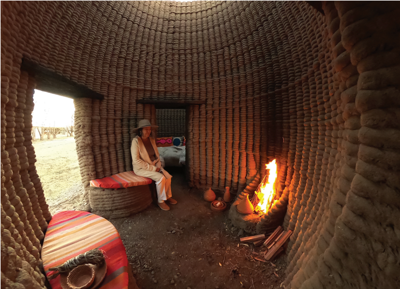
7 The central hearth space of Casa Covida with integrated, printed furniture, including space for sleeping in adjacent room.
