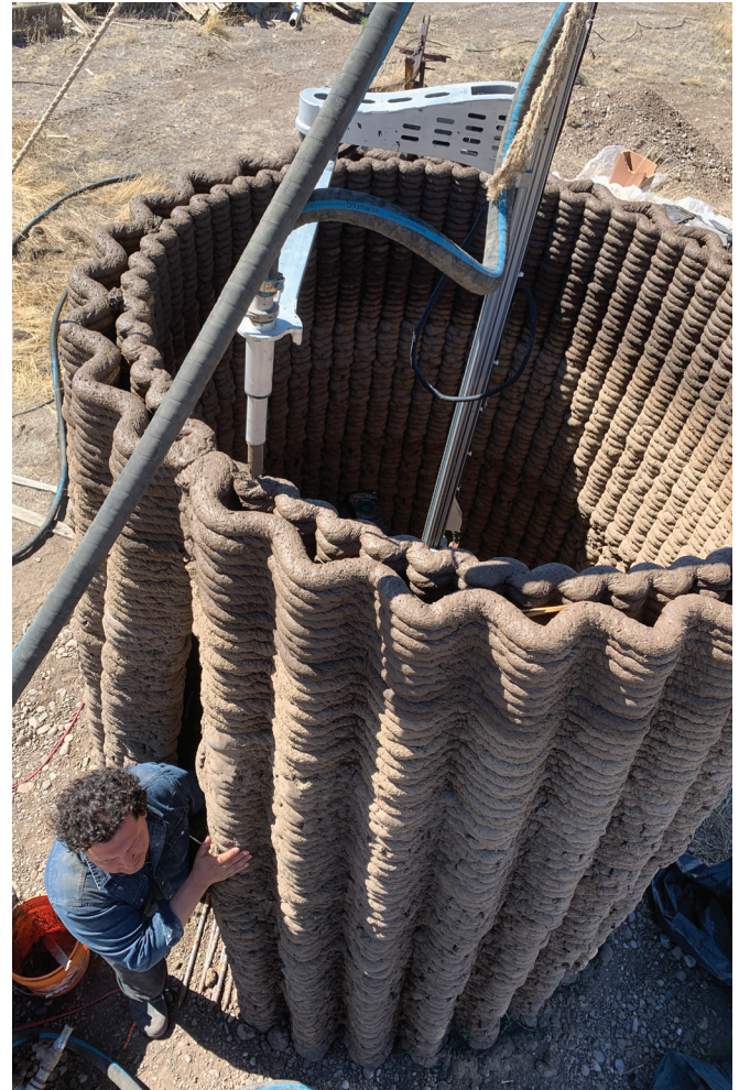
4 The first doubly-walled prototype frustrum space under construction..
