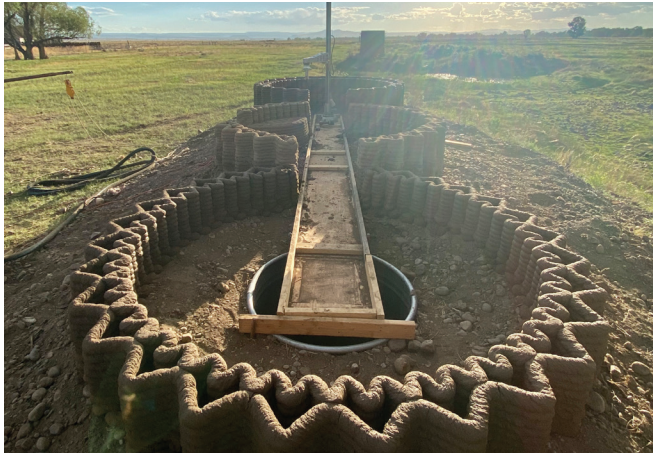
2 A static 4th axis constructed on site facilitates multiple printing positions.
