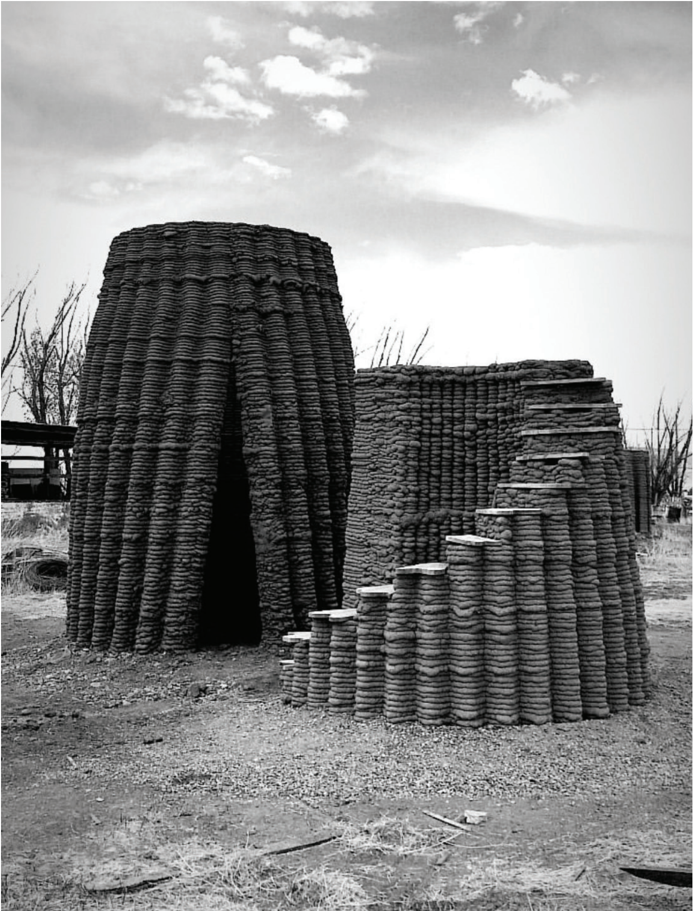
5 Two full prototypes exploring the integration of functional apertures and stairs.
