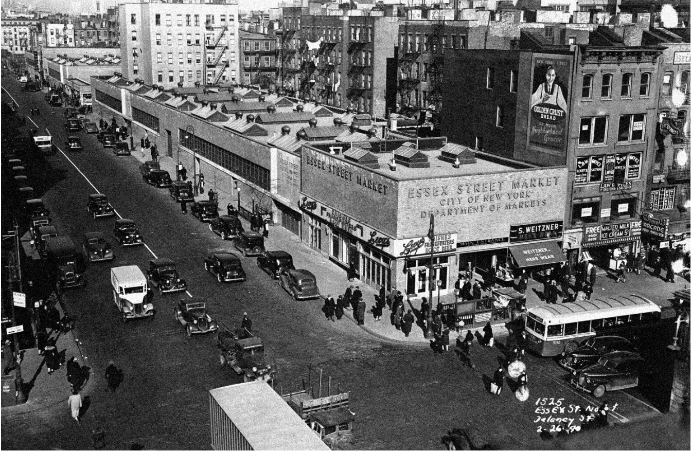
Figure 29. Historical Essex Street Market Building. Image credit: NYC Municipal Archives, Courtesy of Essex Market.
