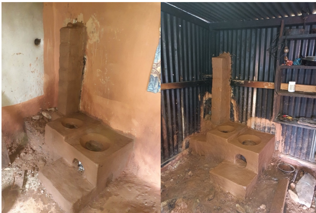
Figure 39: Completed M-ICS in Salambu
