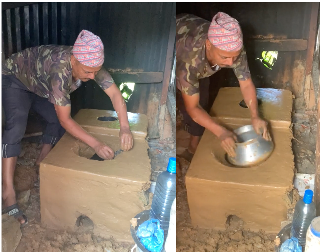
Figure 38: Dilli Dai adding chamfer to potholes for tight seal
