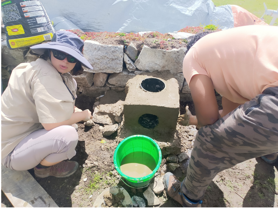
Figure 43: Left to right - Robyn Richmond and Rahul Paramane constructing the prototype one-pot stove
