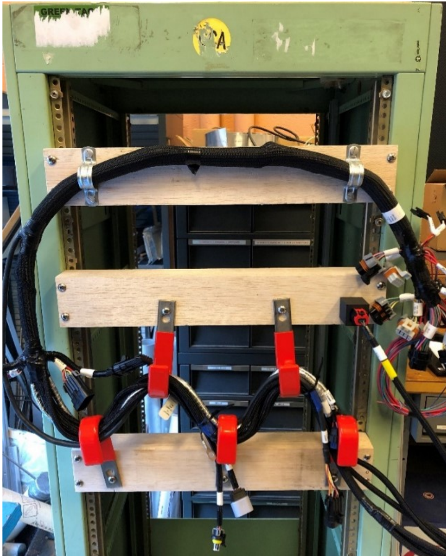
Figure 2-1: after a subject had finished the Manipulation Experiment. On the bottom half of the wire harness are the zip ties that were used to tie the branched ends of the wire harness (Step 1 and 2). On the top half of the mock electrical cabinet are the u-brackets used to screw the wire harness on the mock electrical cabinet (Step 3). The red hooks were placed so that the subjects could route the wire harness (Step 4). A 3D printed socket appears above the right most red hook for subjects to plug the wire harness connector into (Step 5).
