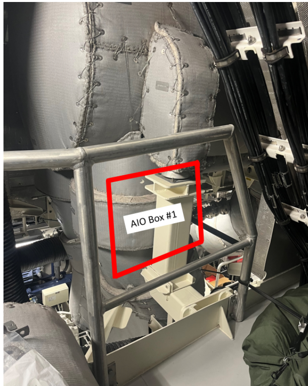
Figure B.2: Location to mount the STBD side AIO Box
