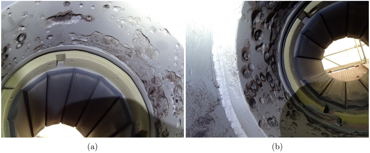
Figure 2.3: Stern tube of USCGC Richard Dixon after sandblasting[23].
