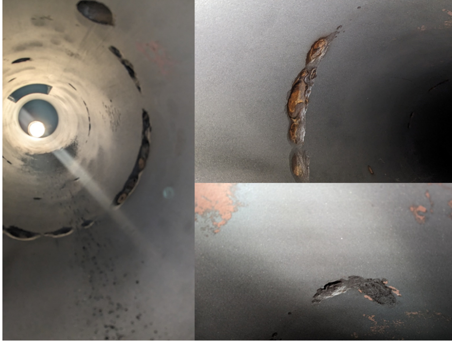
Figure 2.5: Deep pitting in the stern tube of USCGC Charles Moulthrop [24].
