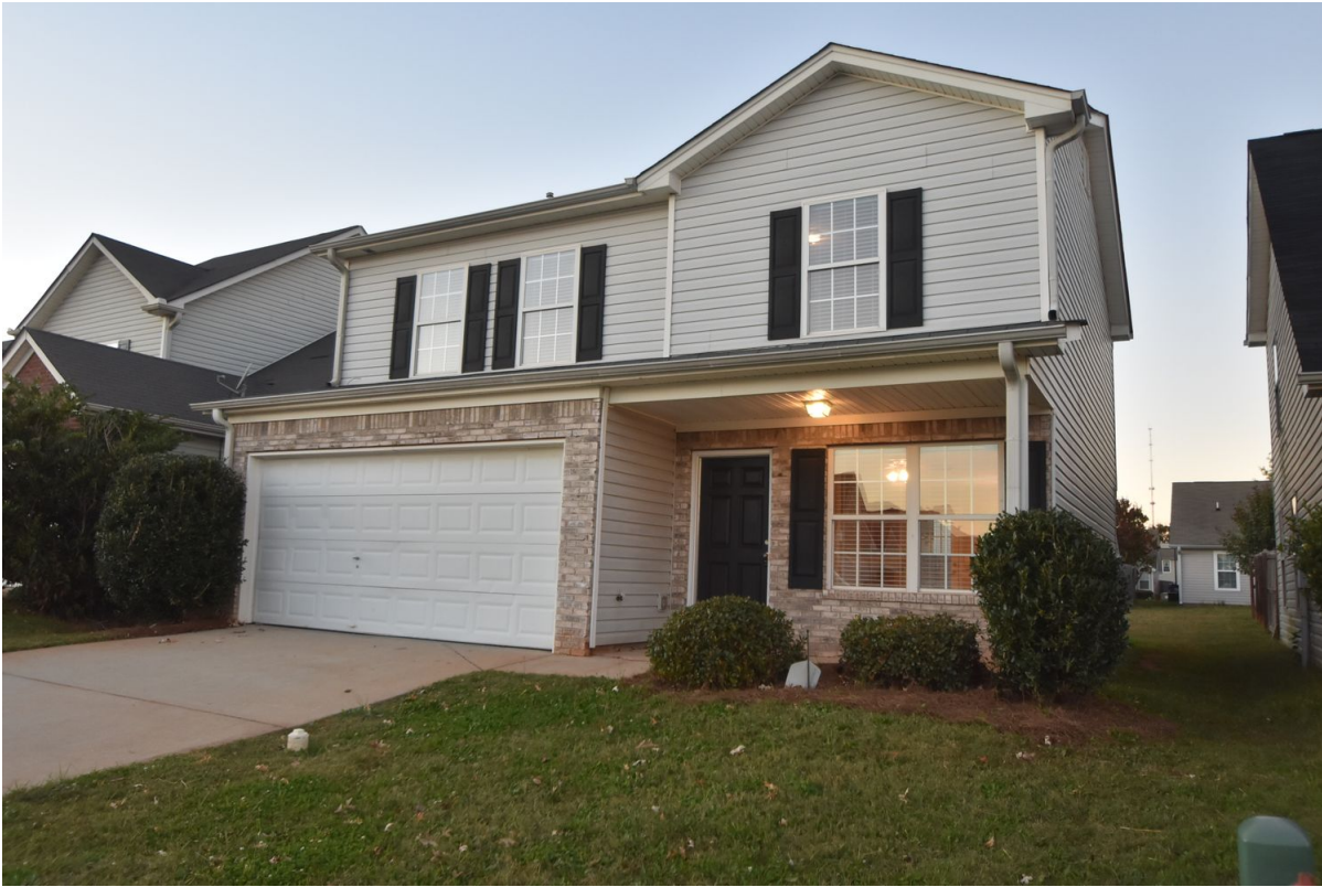
FIGURE A.6: HOUSE EXTERIOR IMAGES
