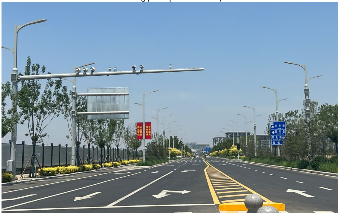
Figure 31. Gantry-mounted cameras and 5G-enabled sensors mounted on lampposts line the newly finished roads of Qidong District (Author, 2023)
