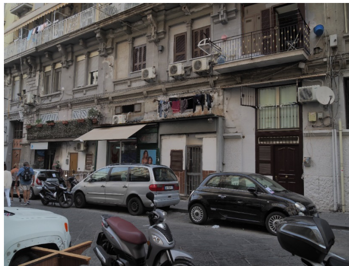
Fig. 39 - Late-nineteenth-century building in Naples ( Via Forcella ) where a formally planned space is informally subverted to meet the needs of residents, resulting in the creation of ground-floor residential units, arbitrary opening of balconies, and blocked-up windows. Photo by author (September 2021).
