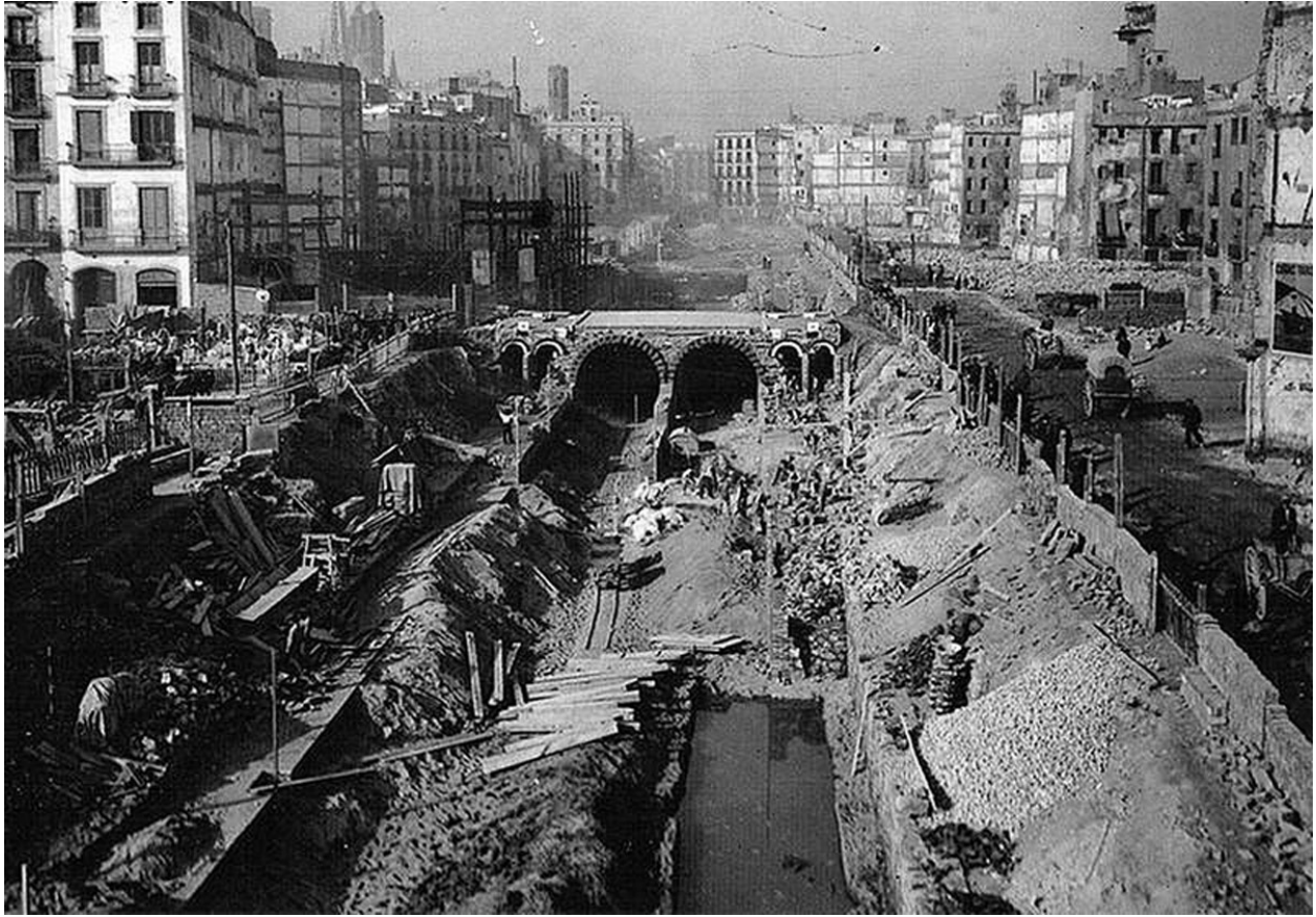
Fig. 27 – Construction works in Via Layetana (1912). Source: Author unknown (Wikimedia Commons).
