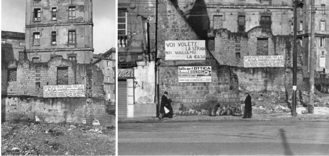
Fig. 73 – Images from the 50s during the construction of the water-facing highway of Via Marina . On the right, the large poster includes the following sentence: “You want the road; we want a home.” – 1950s image of Via Marina . Source: Archivio Iannello .
