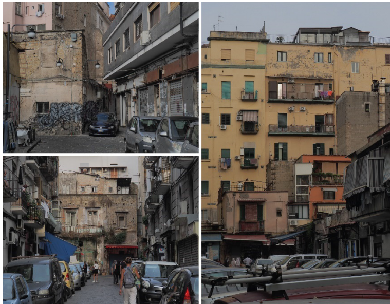
Fig. 41 – Poorly maintained semi-abandoned buildings in Naples. Photos by author (September 2021).
