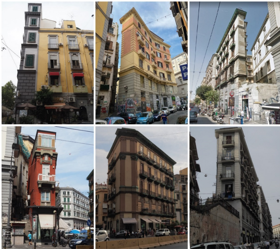
Fig. 40 – Repertoire of thin facades masking the city of Naples. Photos by author (September 2021, June 2022, December 2022).
