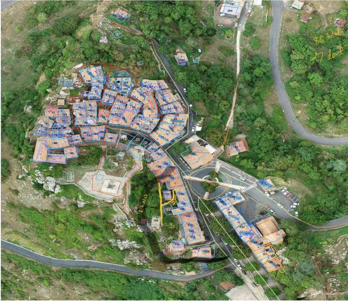
In-process map of Guadagnolo, with the facades of each building numbered and estimated time it takes to complete a portion of the visual survey.
