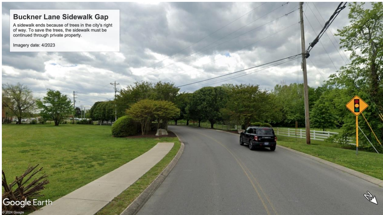
Figure 23: Street view of sidewalk gap on Buckner Lane
