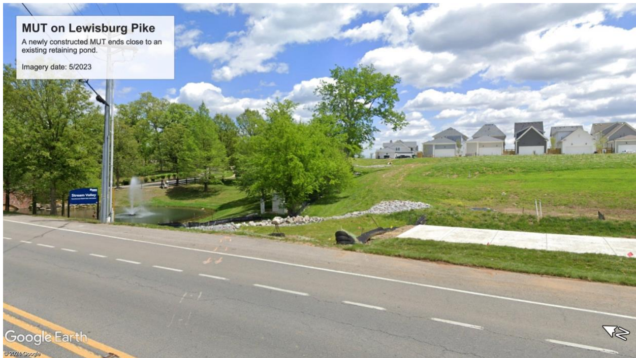
Figure 16: Street view of MUT on Lewisburg Pike
