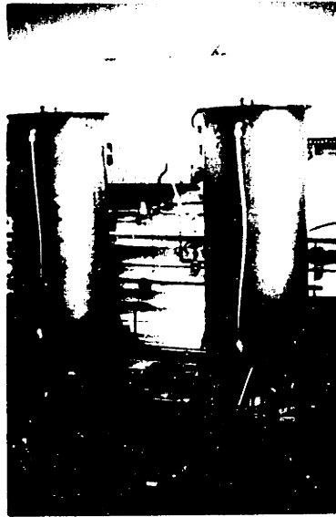
Figure 5.4 Solution Storage and Mixing System- Titanium Tanks
