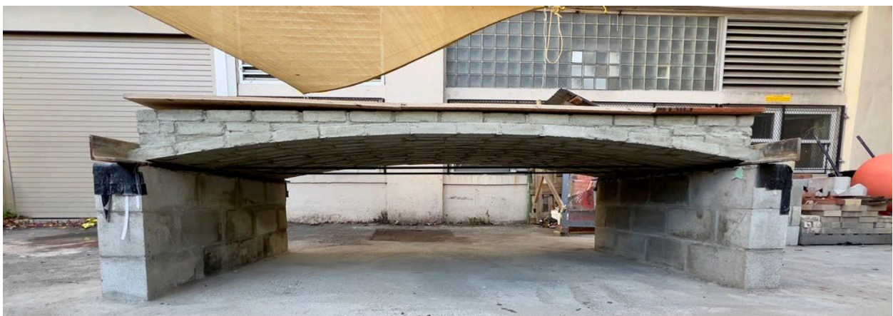
Figure 39: Completed vault floor prototype elevation view
