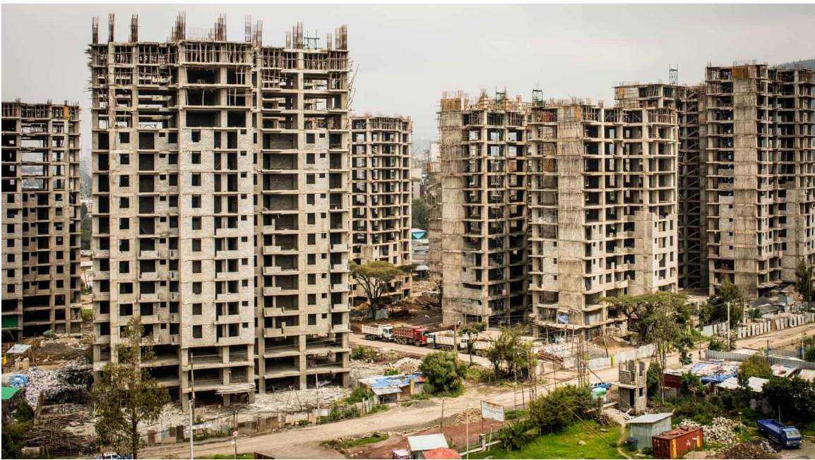
Figure 56: 40/60 condominiums under construction on outskirts of Addis Ababa [Charlie Rosser, 2017]
