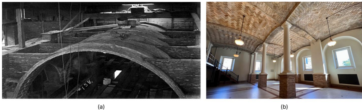
Figure 8: (a) Ribbed barrel-vaulted floor/roof system in Boston Public Library (Ochsendorf, 2010); (b) Shallow double curved thin tile vaulted roof system in Boston Public Library (1895)
