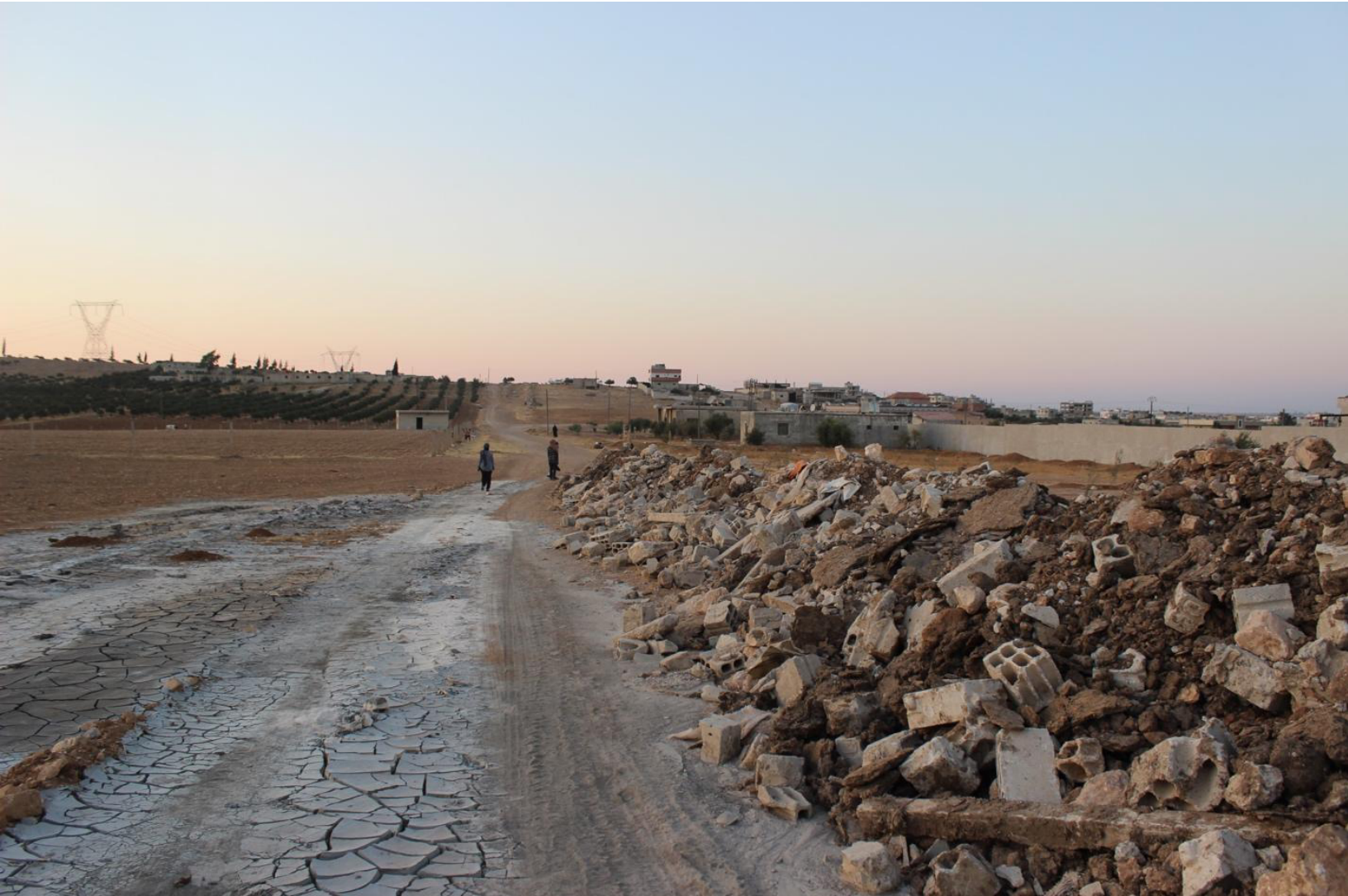
Fig 5. Rubble, Soil, and Construction Waste Line the Street in Nasib, 2021
