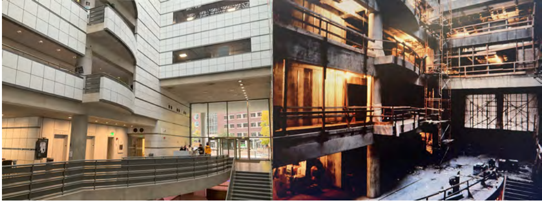
Figure 13: E15 after and before
