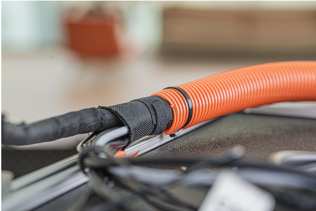
Figure 3.13: The system umbilical contained a bundle of fluid lines as well as electrical connections, it was sheathed and shielded to protect and isolate the contained interconnections. Photograph system umbilical as is breaks out into different lines at the distal end
