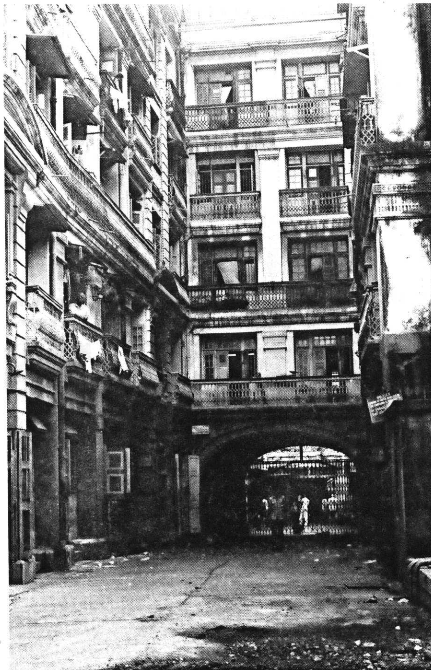
PHOTOGRAPH: The court surrounded by dwelling; the back entrance is kept closed most of the time
