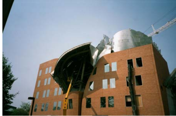
B. Concrete form work – Weatherhead School
