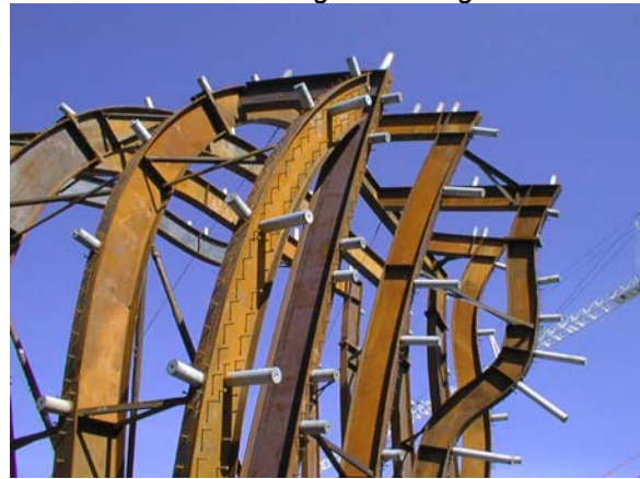
D. Rib assembly on site
