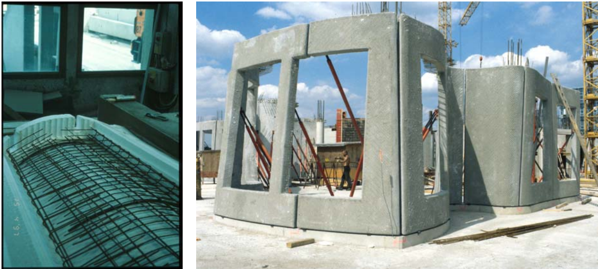
Figure IV-4: CNC fabrication of cast concrete (Dusseldorf)
