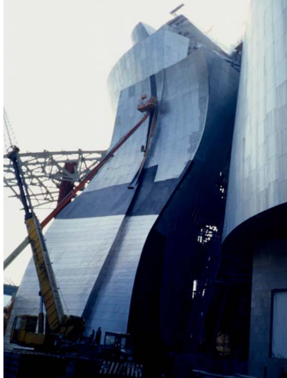
Figure IV-9: Macro and element scale sheet forms (Bilbao)
