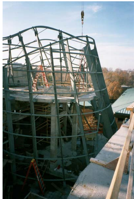
Figure VI-28: Stick and pipe structural system
