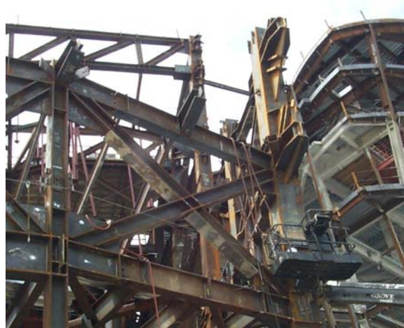
Figure III-23: Connection geometry on DCH
