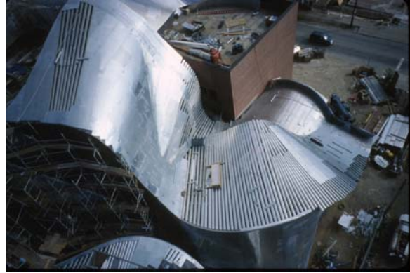
Figure VI-30: Back pan on hat channels
