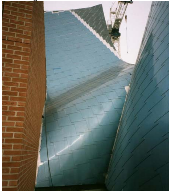
Figure VI-32: Shingled developable form
