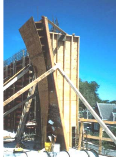
B. Template cut formwork
