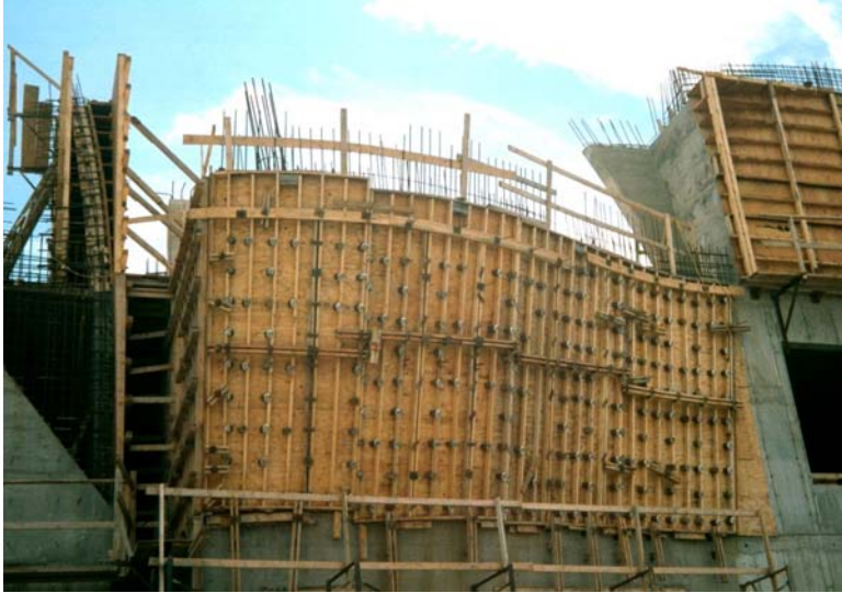
A. Developable surface formwork
