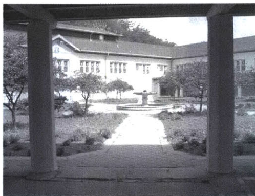
fig. 23 Fuller Park field house courtyard.
