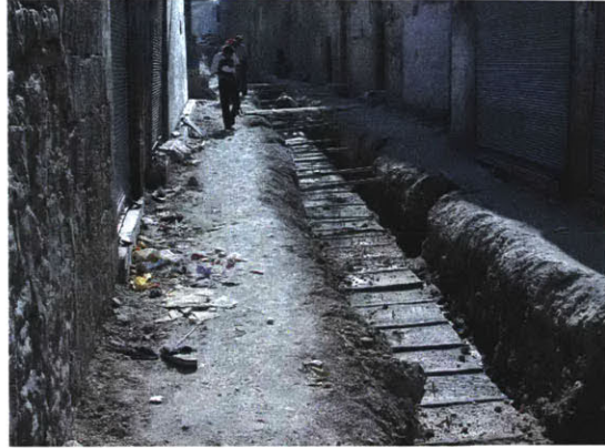
Figure 17. Upgrading sewer and water infrastructure
