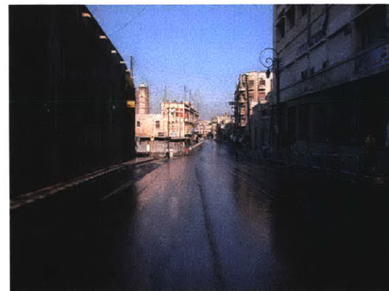
Figure 8. Four lane thoroughfares in the old city as a result of master planning
