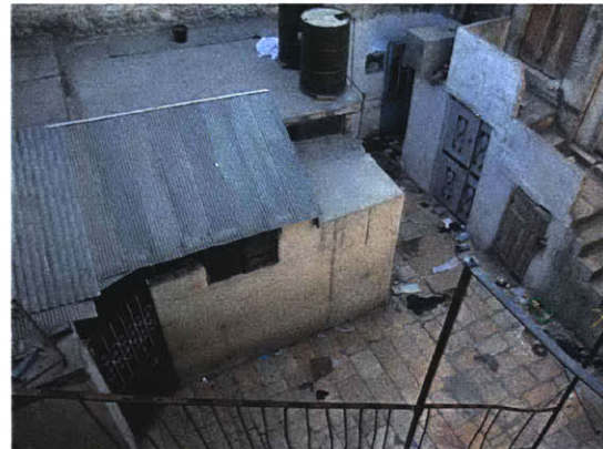
Figure 11. Closed structure constructed inside courtyard
