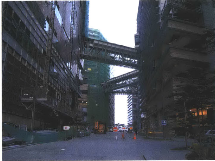
Fig. 3.6 Image of Biopolis under construction. Photograph by the author March 2004.
