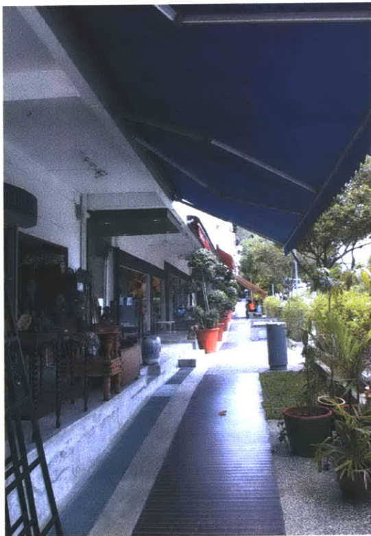
Fig. 5.3 View of renovated arcades at Chip Bee live-work apartment complex. Photograph by the author March 2004.
