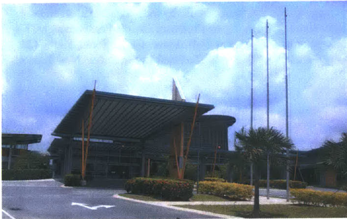
Fig. 4.8 The Cyberjaya Smart Command Center is intended to act as a coordinating center for the utilities serving the entire development when the park reaches higher capacity. Photograph by author March 2004.
