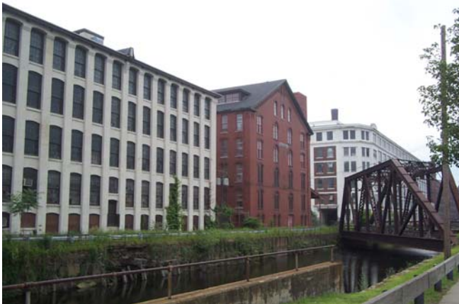
View of the Duck Mill, Pemberton Mill and Washington Mill seen from the North Canal.
