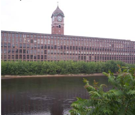
View of the Ayer Mill and clock tower.
