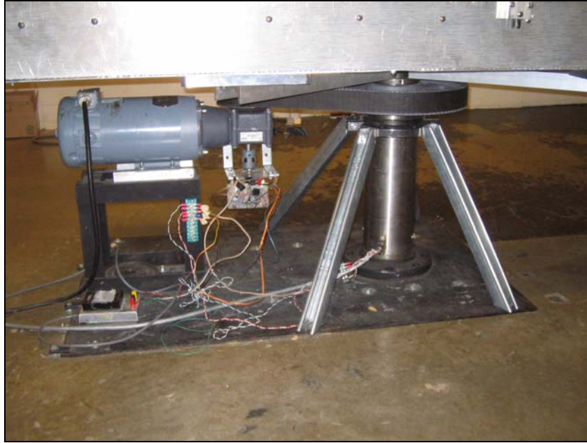
Figure 3.9. View of the new stabilizing tetrapod.
