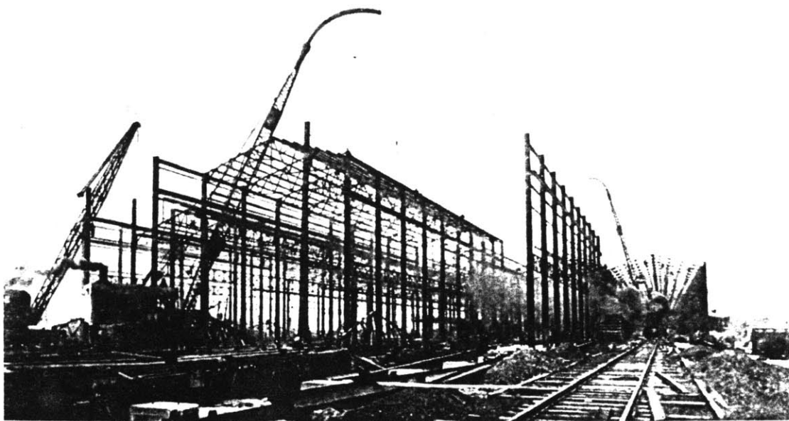
Ford Shipbuilding Plant. Job #847. (1919) Dearborn, Michigan
